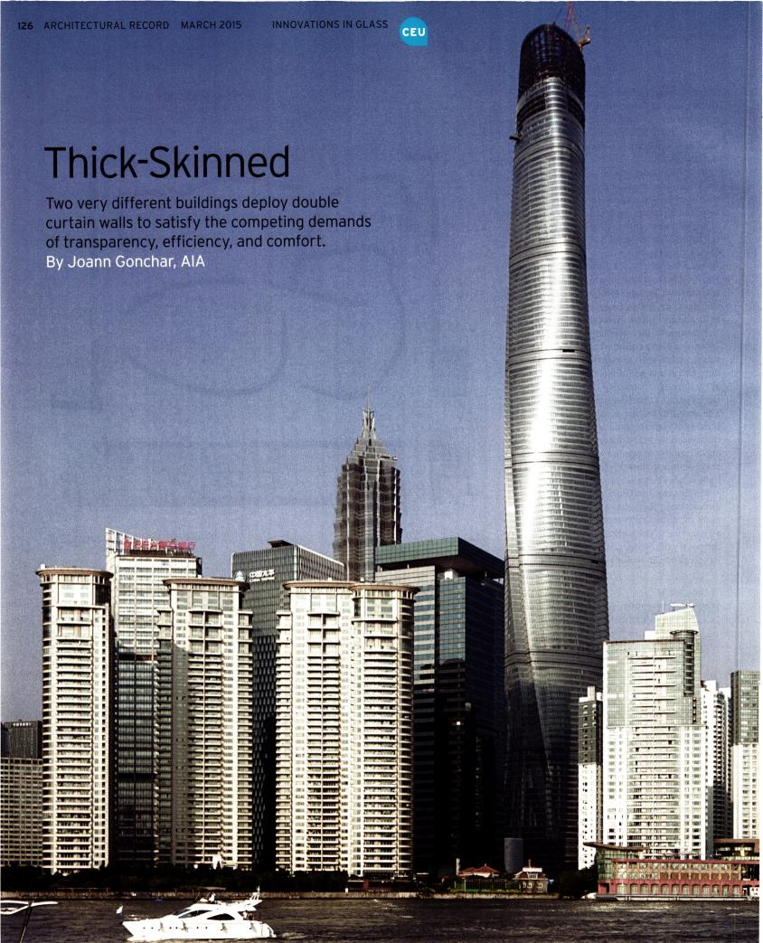
THE DOUBLE-SKIN curtain wall-an enclosure system that consists of two facades separated by a cavity-has long been a popular approach to all-glass buildings in Europe, in part due to higher energy prices and tougher energy codes there. But such walls have begun to proliferate in other parts of the world as a way to satisfy the sometimes competing goals of transparency, efficiency, and occupant comfort.
