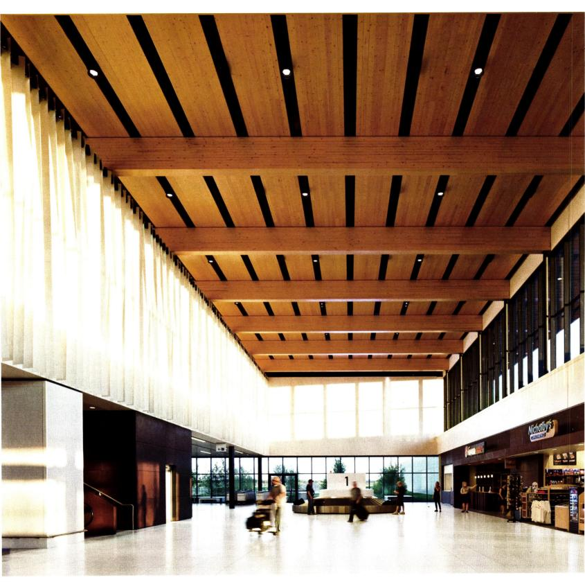
MATERIAL CUES The engineered-wood ceiling is one of the longest continuous spans of CLT in North America (above). A wall clad in white laminated-MDF tile provides an acoustic buffer opposite the metal-slat "curtain" (opposite, left). Information screens and receptacles are discreetly embedded in terminal walls (opposite, right).
