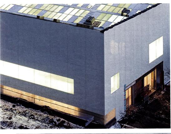
high, each one supporting the one above it and transferring dead loads to the foundation. The 140 panels were fabricated in Germany by Thiele Glas. German facade contractor MBM Konstruktionen coordinated their assembly at Thiele's factory, affixing aluminum supports to the back of the glass with structural silicone. These coat-hook-type elements fasten onto U-channels mounted on the building's exterior sheathing, facilitating installation.
