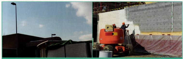
Rigid foam boards (left) come in standard sizes and need to be cut and fit into wall assemblies. Spray foam insulation (right) is directly applied to the appropriate surface of the wall assembly in the quantity needed.
