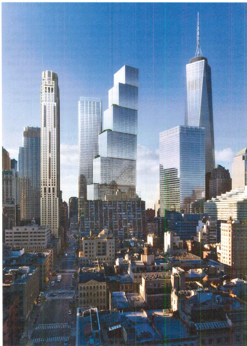
BIG’s design of 2 World Trade is made up of seven staggered boxes. Catered to a modern media company, each volume will function as its own building and include double-height atria, views between floors, and access to generous terraces.
