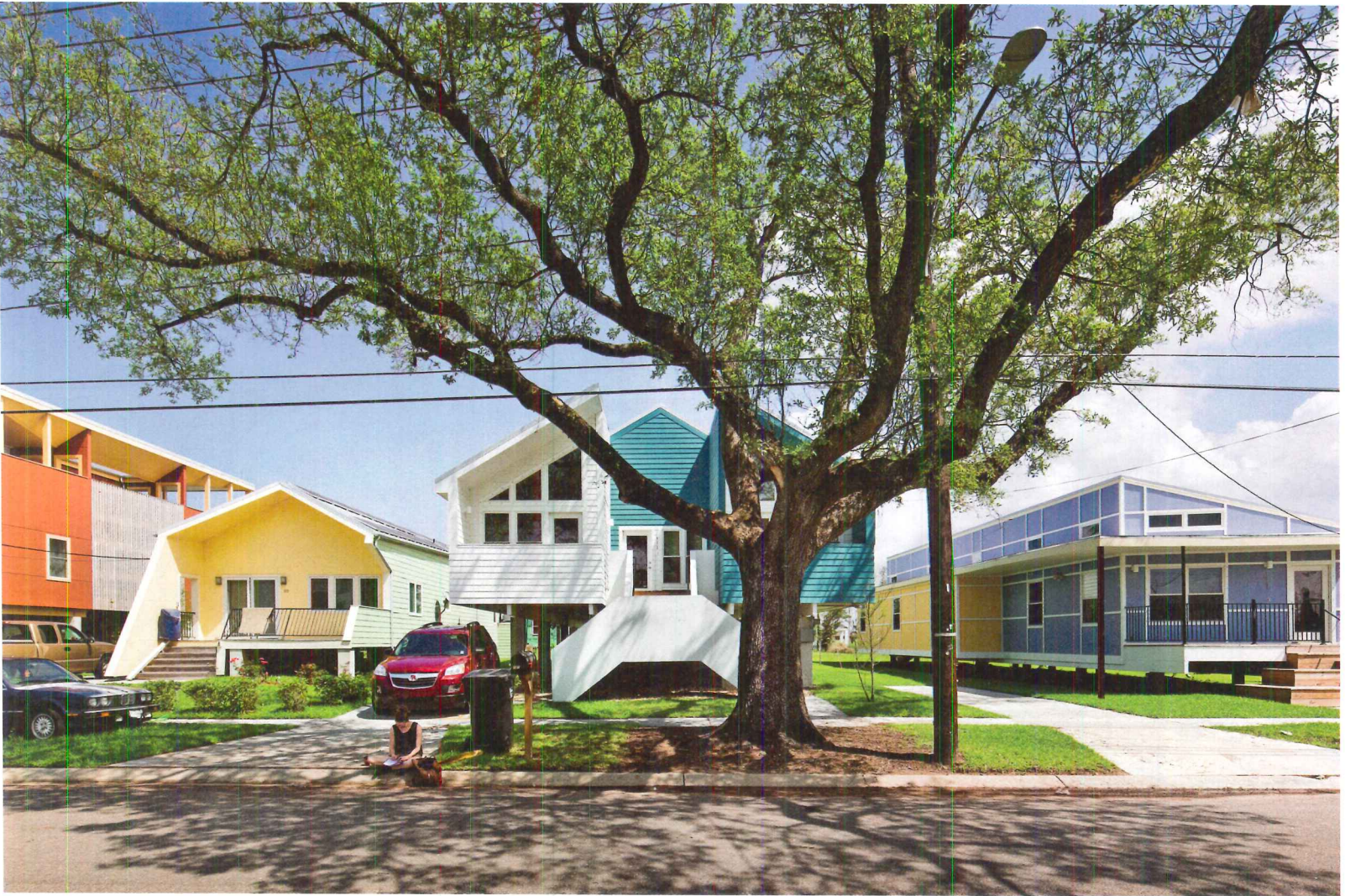
CLOSER TO EARTH Houses built by Make It Right in the Lower Ninth Ward illustrate how risk assessments have changed in recent years. The Hitoshi Abe duplex (center) completed in 2009 was built a full floor above grade to survive a catastrophic levee break. Newer houses are more modestly elevated, under the assumption that the nearby levee will hold.
