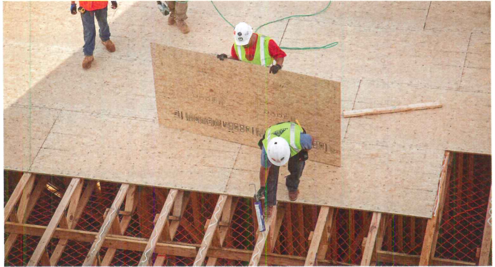
High-performance engineered wood panels maintain strength and stiffness values, even after exposure to elements throughout construction, which ultimately helps provide consistently quiet, stiff finished floors.
