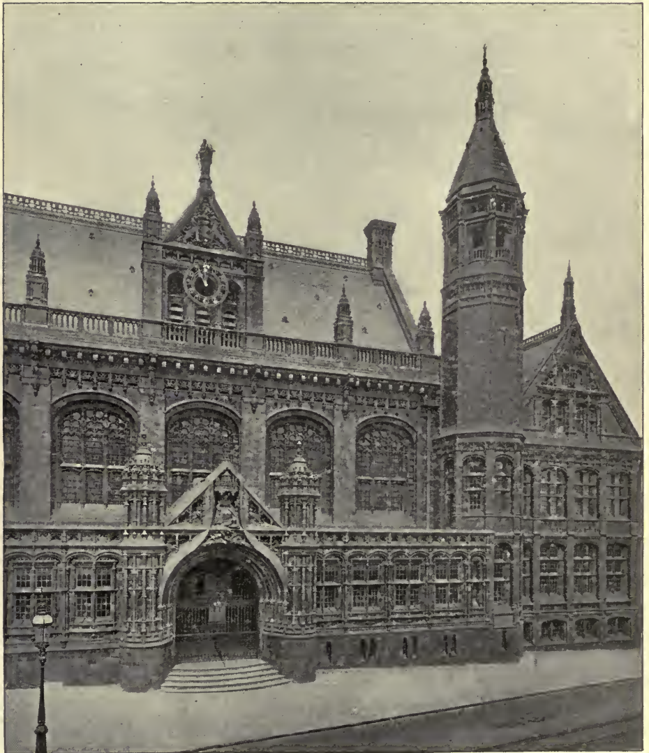
EXTERIOR OF BIRMINGHAM LAW COURTS.
