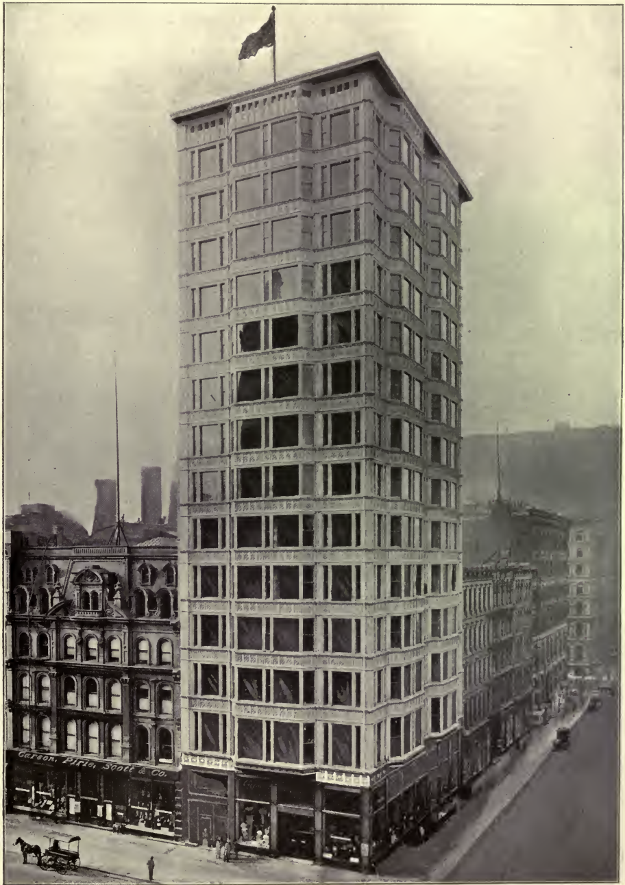
RELIANCE BUILDING—CLOSED IN NOVEMBER 8.
