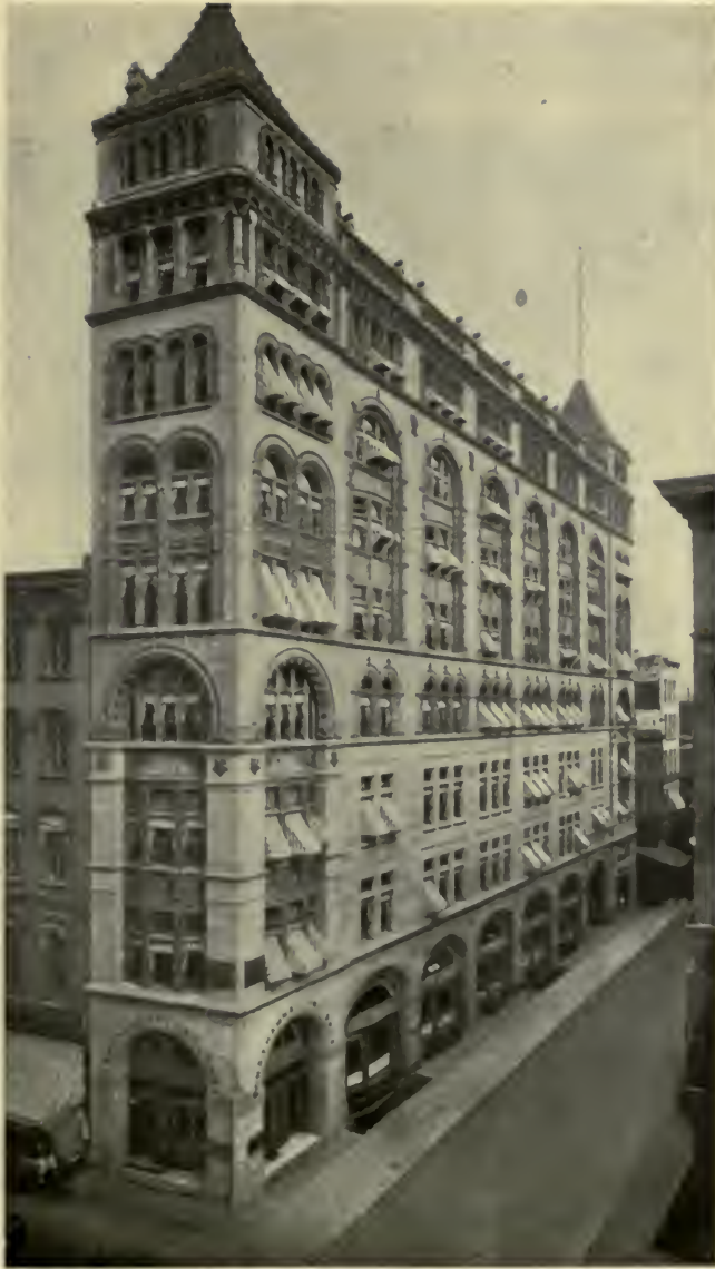
CORBIN BUILDING—1888-1889. Broadway, Northeast Corner John Street. F. H. Kimball, Architect.
