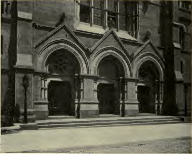
Entrance, Emanuel Baptist Church.—1885.
