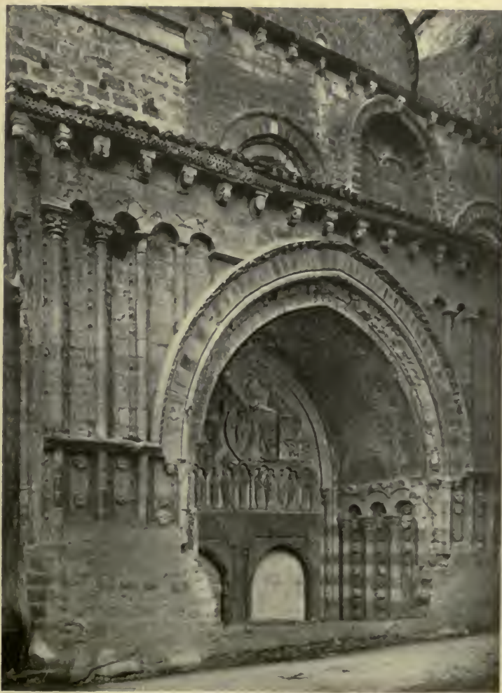
North Portal, Cahors Cathedral.
