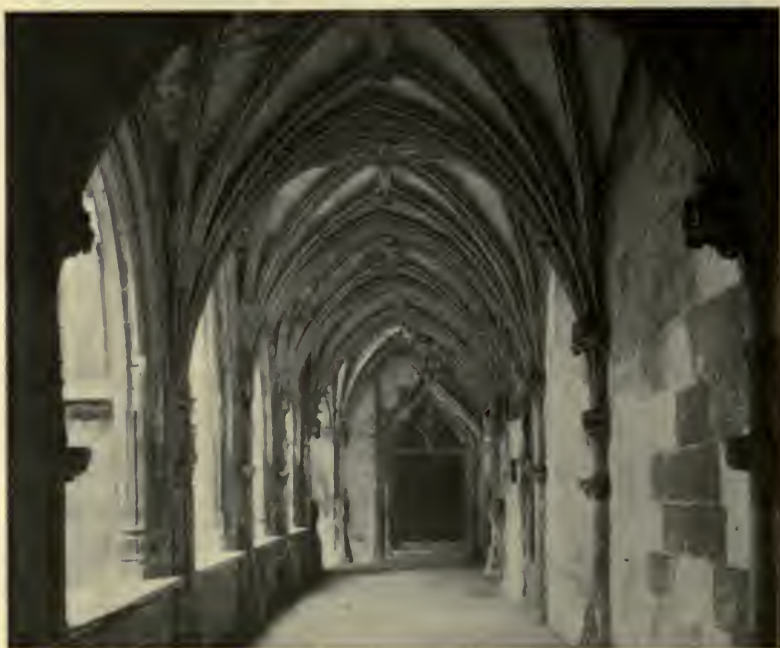
Cloisters, Cahors Cathedral.
