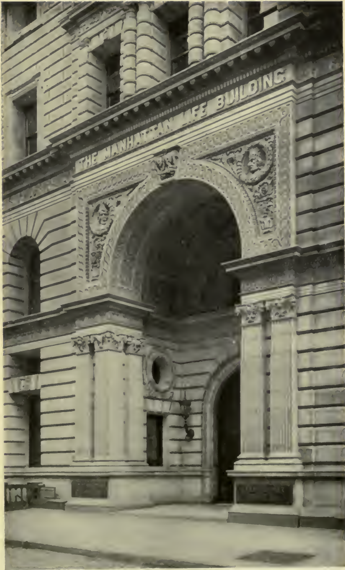
MANHATTAN BUILDING. Broadway Entrance. Kimball & Thompson, Architects.
