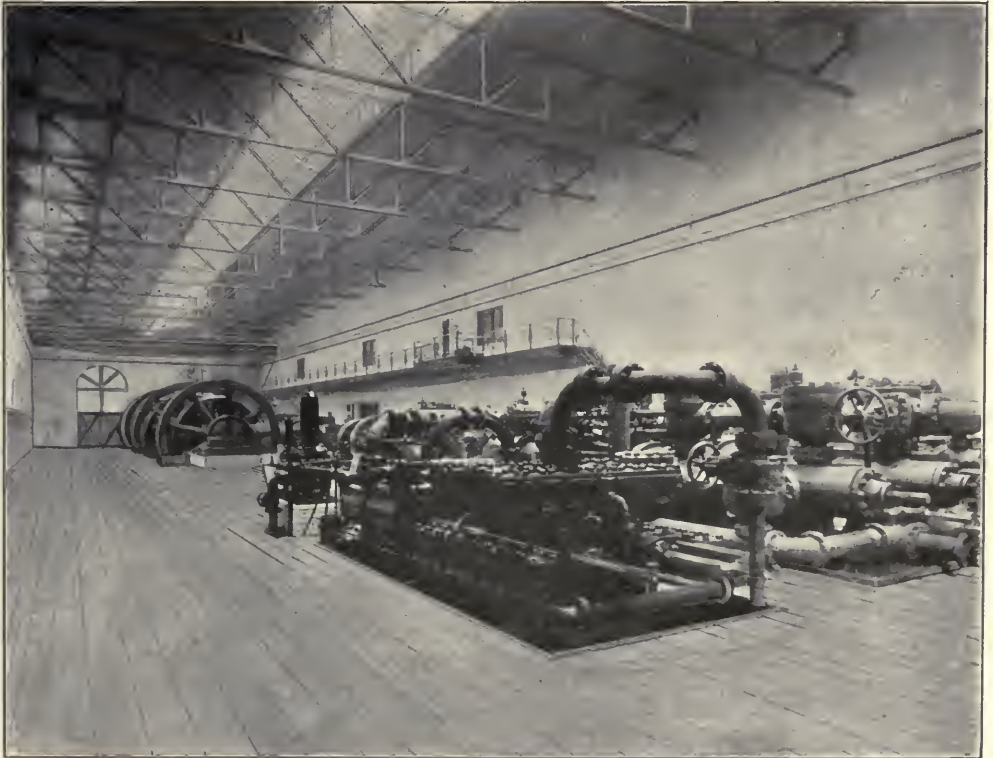
ENGINE AND PUMP ROOM—SEARS, ROEBUCK & CO. BUILDINGS.
