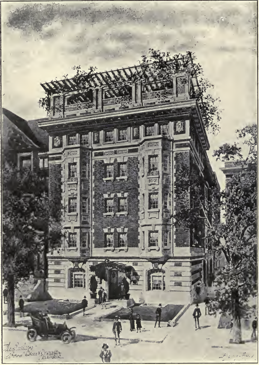
"THE BACHELOR" APARTMENT HOUSE.
