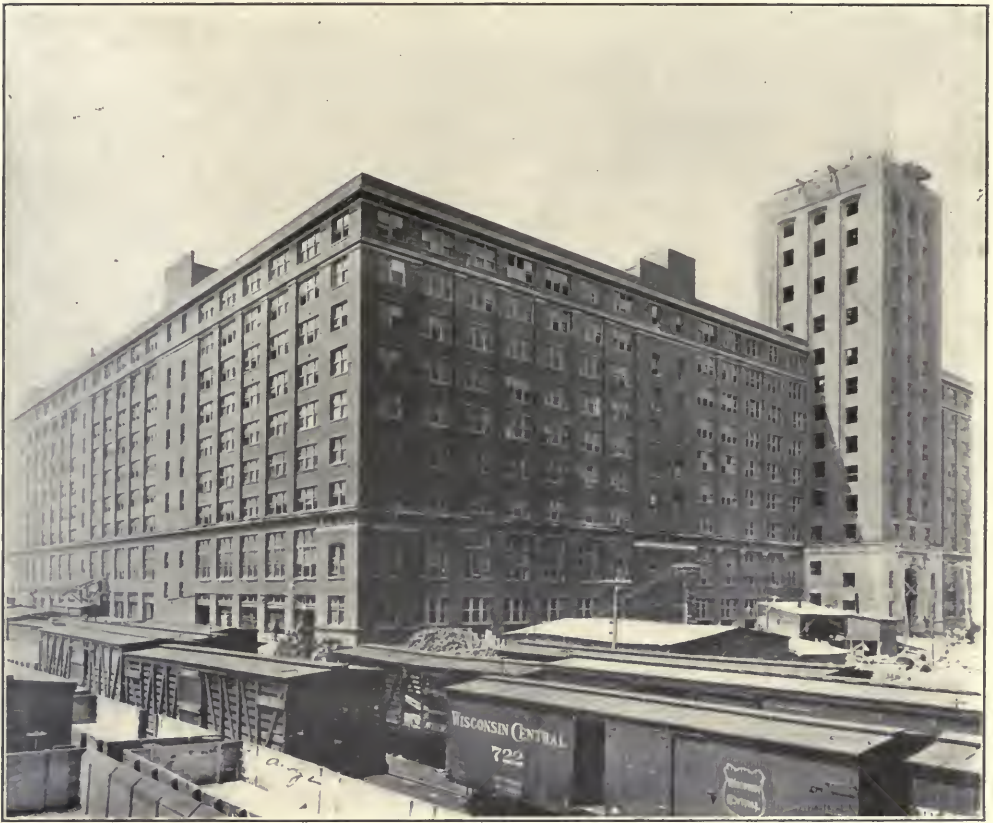
MERCHANDISE BUILDING, LOOKING NORTHWEST—SEARS, ROEBUCK &amp; CO.
