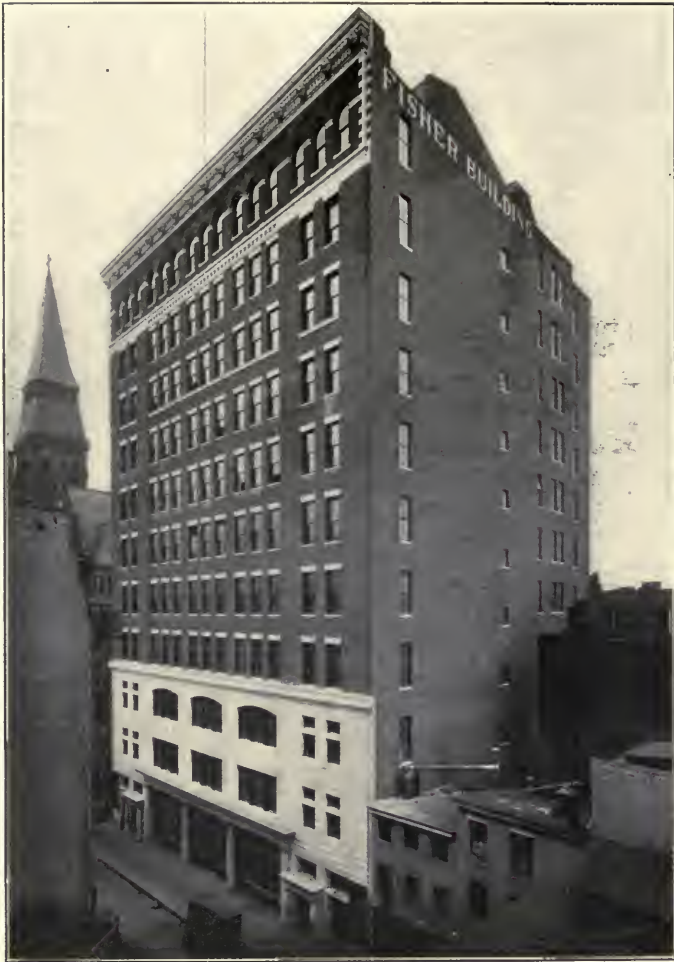
FISHER BUILDING, 97-103 EAST HOUSTON STREET, N. Y. CITY. Cream White Glazed Terra Cotta, Vellum Finish.
