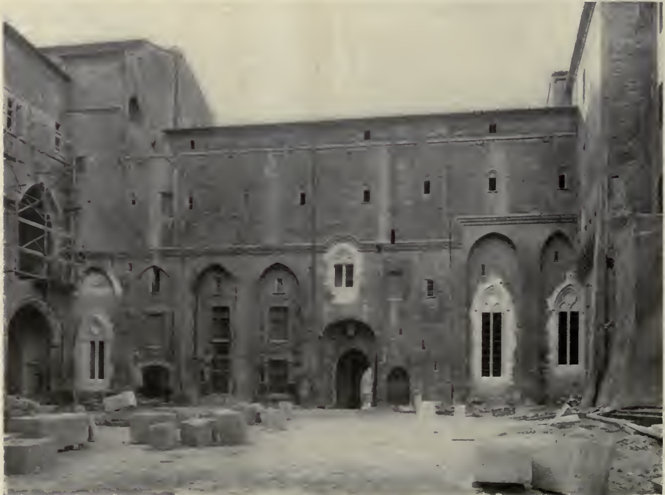
WESTERN FAÇADE FACING COURTYARD.
