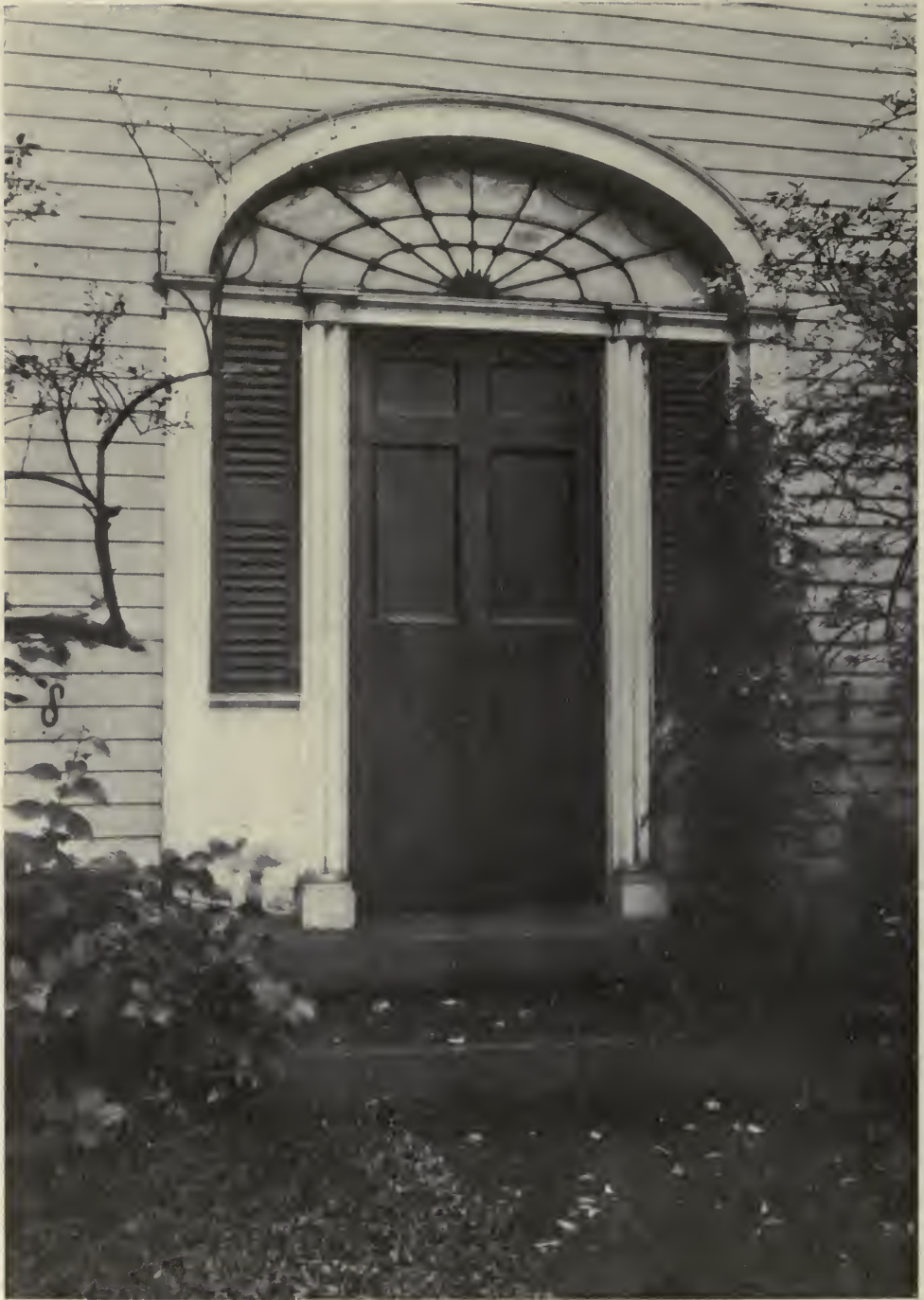
An unpretentious flat doorway on a Deerfield house. Its lines throughout, even to the leaded glass of the fan, are most pleasing; but its distinguishing feature is the engaged double colonnette each side of the door, with its two members egg-shaped, not round.
