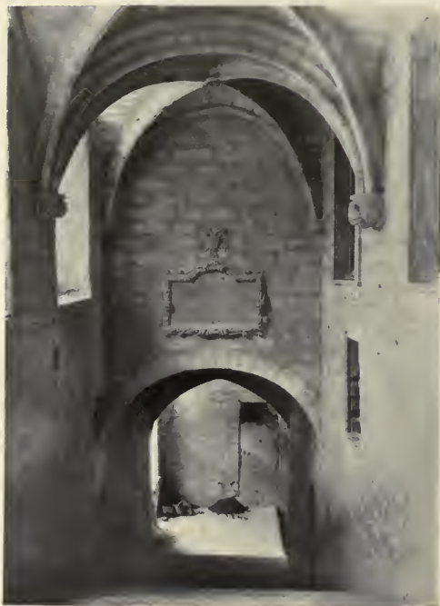
STAIRCASE LEADING TO THE PONTIFICAL CHAPEL OF CLEMENT VII—RESTORED IN 1659.
