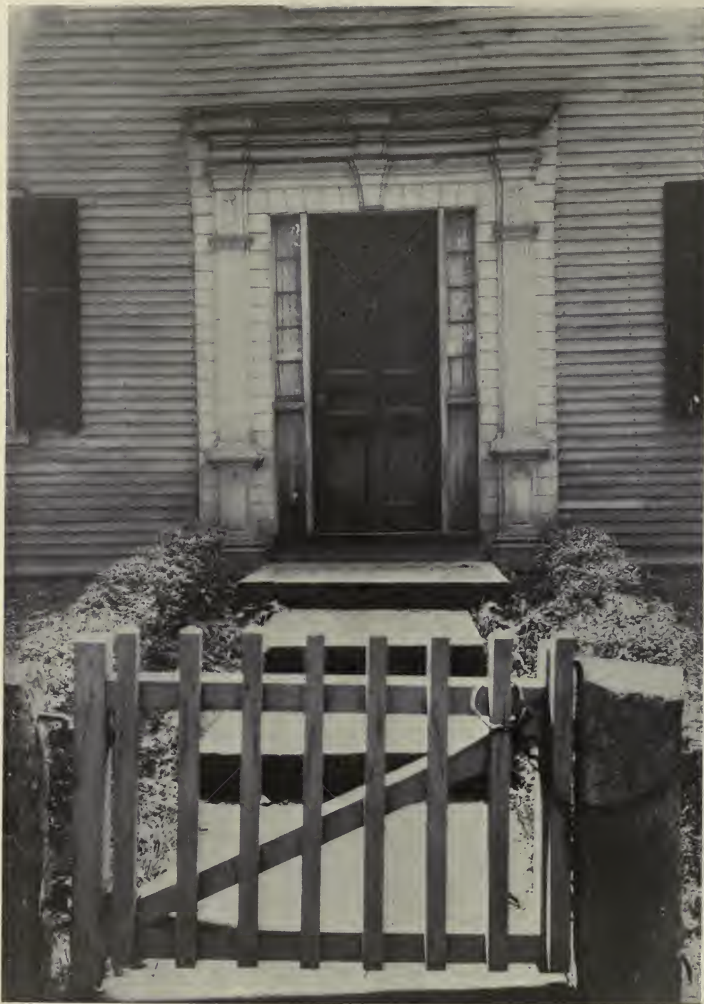
A Deerfield example that is a literal copy in wood of a Georgian stone doorway. Made before Colonial Woodworkers had learned the more graceful and more delicate possibilities of their material; in fact it is early enough to still show a trace of Gothic feeling in the lower panels. It is interpreted with as much naivety and innocence of classic proportions as was its prototype interpreted from the Italian Renaissance. Although of the same date as the house, the door was not built in situ but was ordered separately from some skilled workman and set up intact in the opening left for it.
