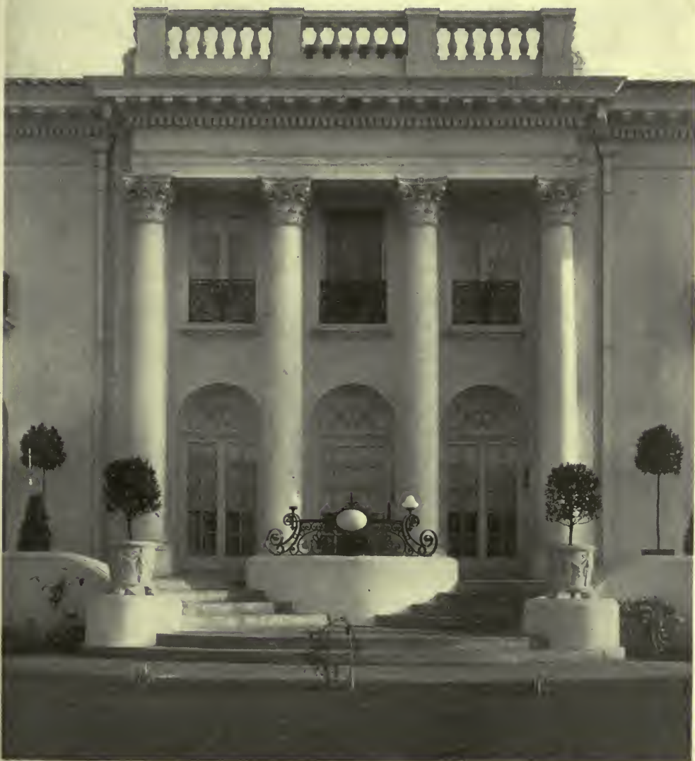
DETAIL—RESIDENCE OF MRS. LOUISE A. DENKER, LOS ANGELES, CAL. B. COOPER CORBETT, ARCHITECT.
