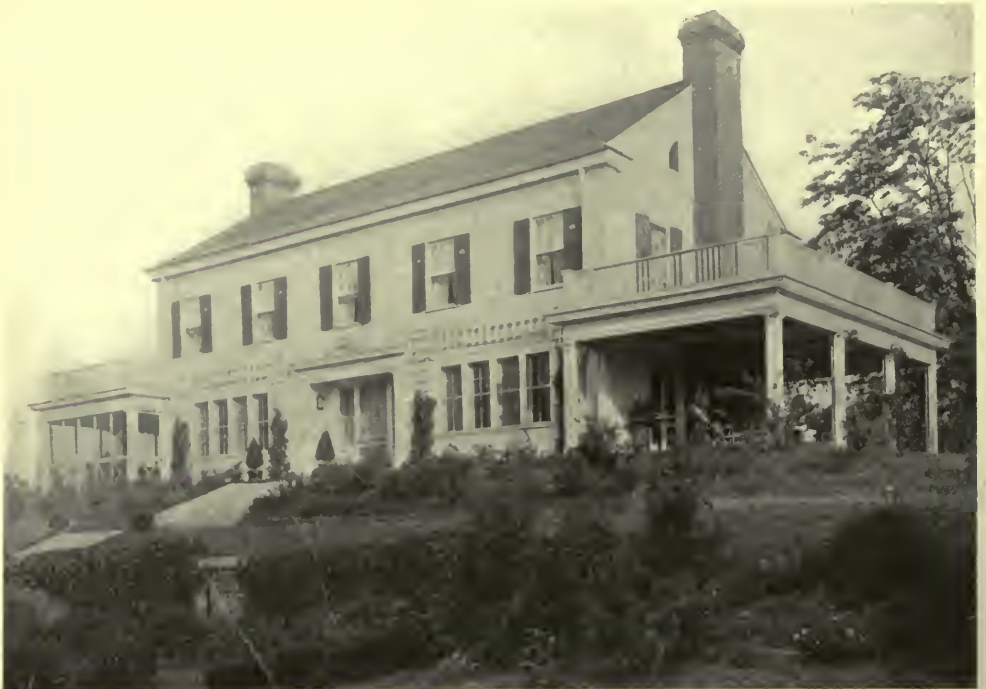
RESIDENCE OF CHARLES M. RANKIN, ESQ., TERRE HAUTE, IND. Otis & Clark, Architects.
