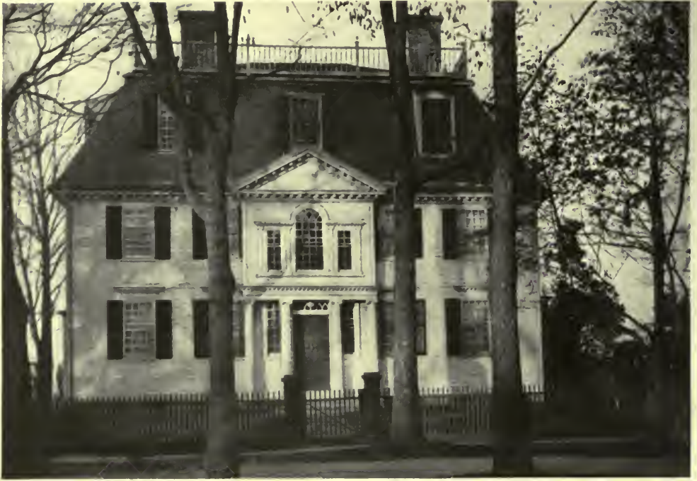
THE SHELDON HOUSE, BUILT IN 1760, LITCHFIELD, CONN. AT THE SIDE IS A "WITCH" DOOR.
