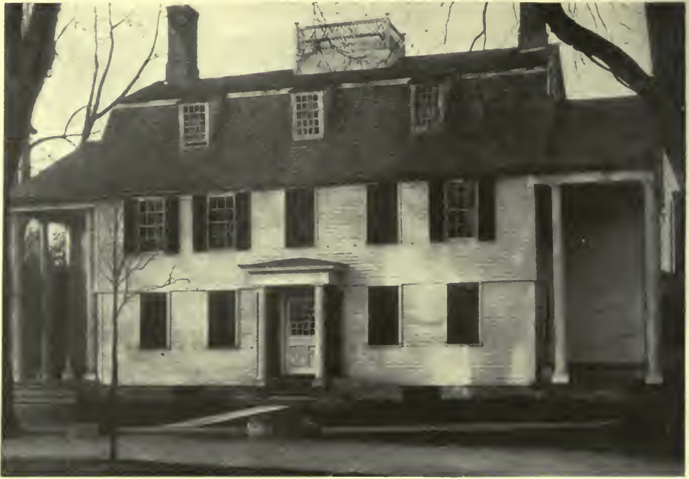
THE TALLMADGE HOUSE, BUILT IN 1775, LITCHFIELD, CONN. THE FRONT DOOR IS OF LATER DATE.
