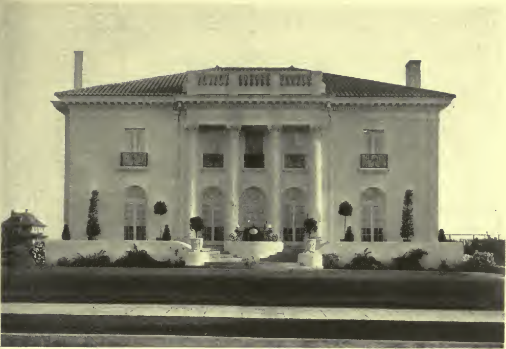
RESIDENCE OF MRS. LOUISE A. DENKER, LOS ANGELES, CAL. B. Cooper Corbett, Architect.
