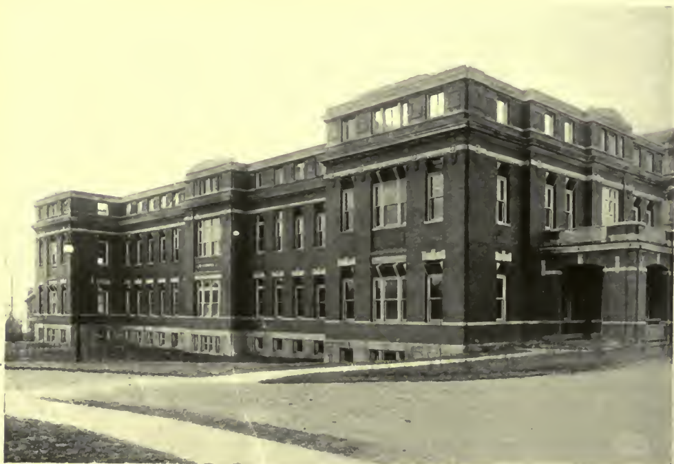
WARD BUILDING "A"—THE NEW GENERAL HOSPITAL, CINCINNATI, OHIO. Samuel Hannaford & Sons, Architects.
