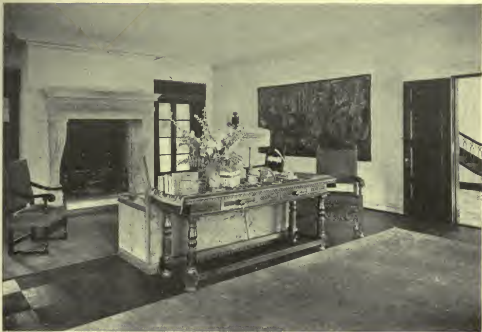
LIVING ROOM—RESIDENCE OF WALTER R. KIRK, ESQ., LAKE FOREST, ILL. Otis & Clark, Architects.
