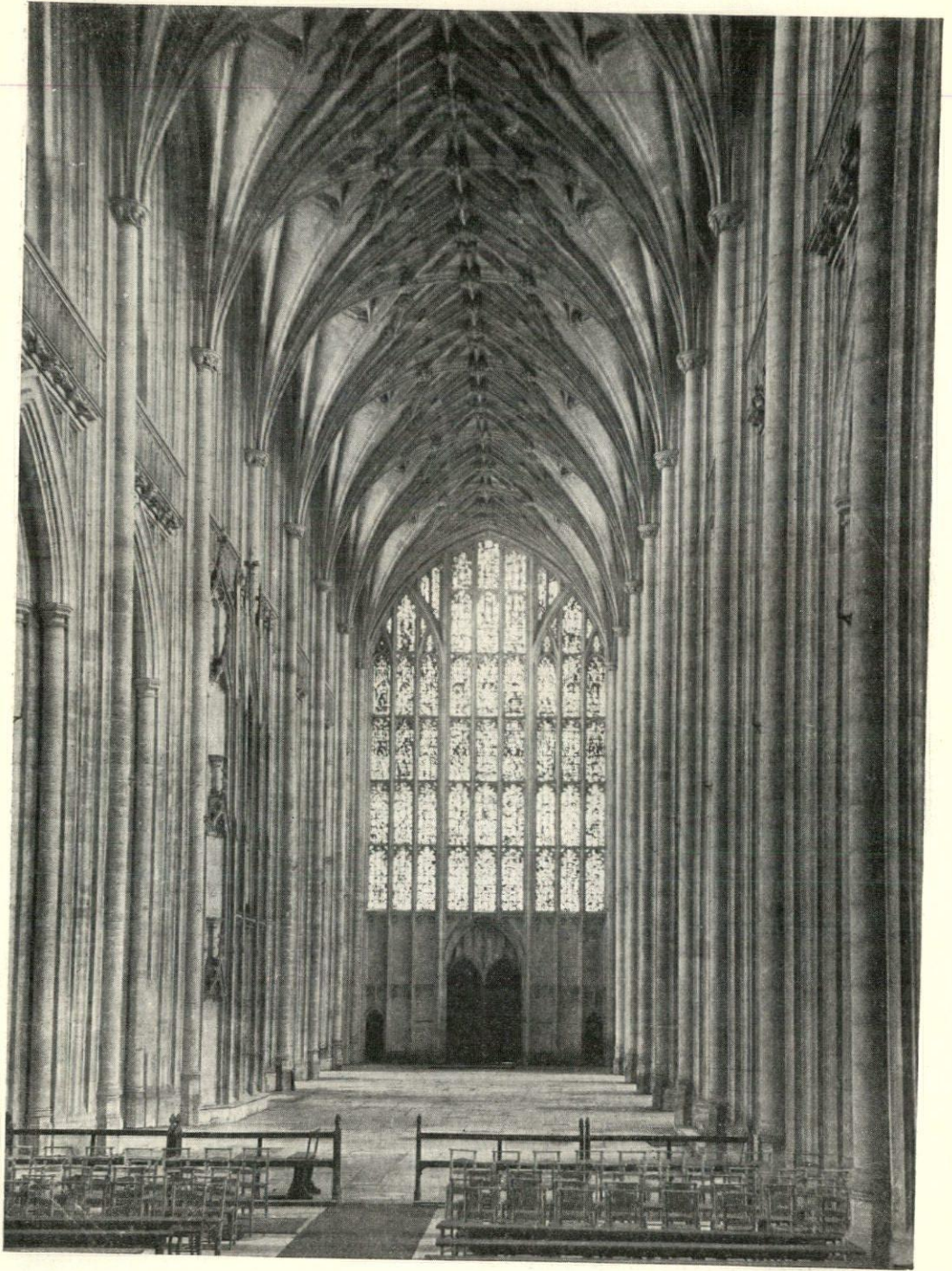
FIG. 4. WINCHESTER CATHEDRAL, NAVE; LIERNE VAULTING, PERPENDICULAR WEST WINDOW; SINGLE CONTINUOUS VAULTING SHAFT.
