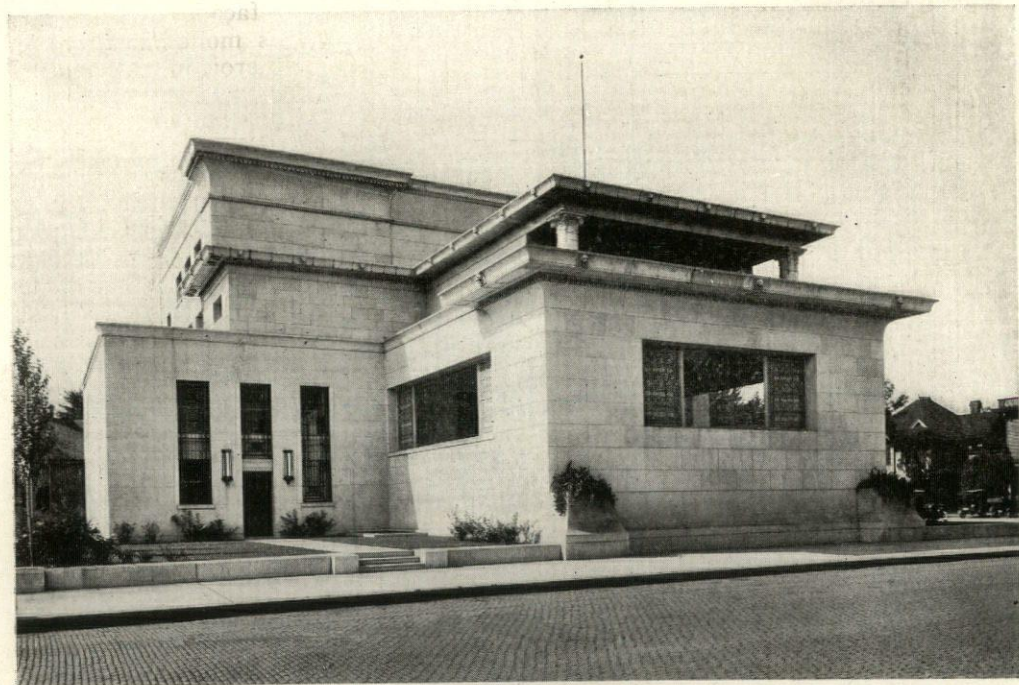
REAR VIEW, FROM THE EAST—WINONA SAVINGS BANK AND WINONA NATIONAL BANK, WINONA, MINN. George W. Maher, Architect.
