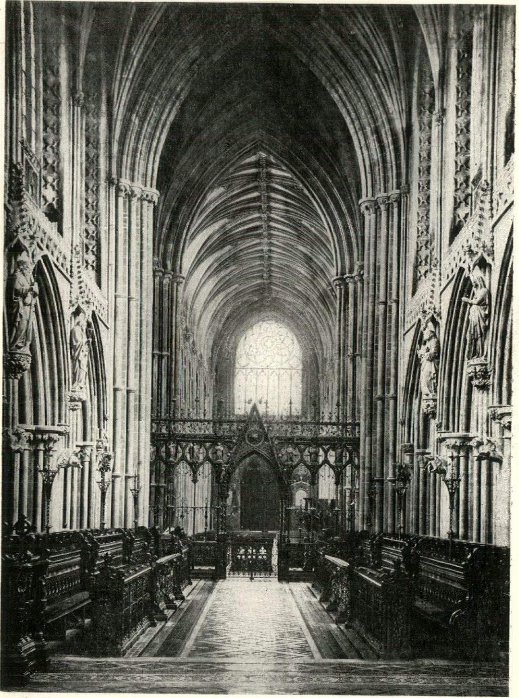
FIG. 3. LICHFIELD CATHEDRAL, CHOIR; TIERCERON VAULT, STRONG RIDGE RIB, RICH INTERIOR DECORATIVE MEMBERING.
