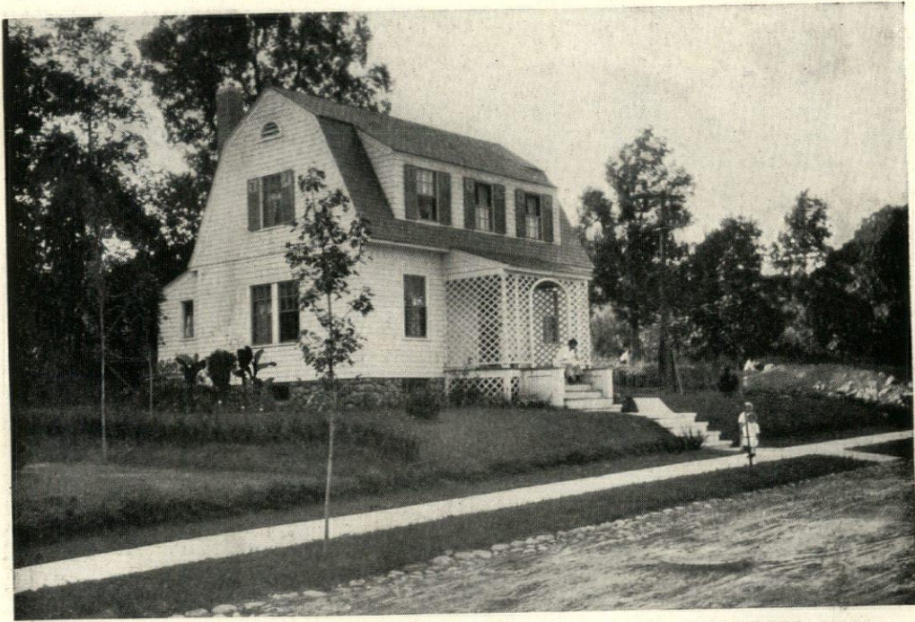
AN INDIVIDUAL HOUSE OF THE SMALLER TYPE—INDIAN HILL, WORCESTER, MASS. Grosvenor Atterbury, Architect.
