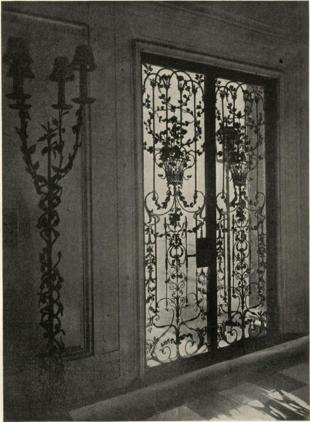
VESTIBULE GRILLES—RESIDENCE OF WILLIAM McNAIR, ESQ., NEW YORK. H. VAN BUREN MAGONIGLE, ARCHITECT.
