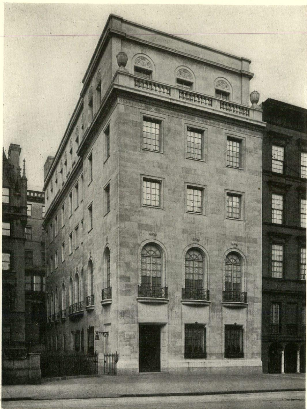
RESIDENCE OF WILLIAM McNAIR, ESQ., NEW YORK. H. VAN BUREN MAGONIGLE, ARCHITECT.
