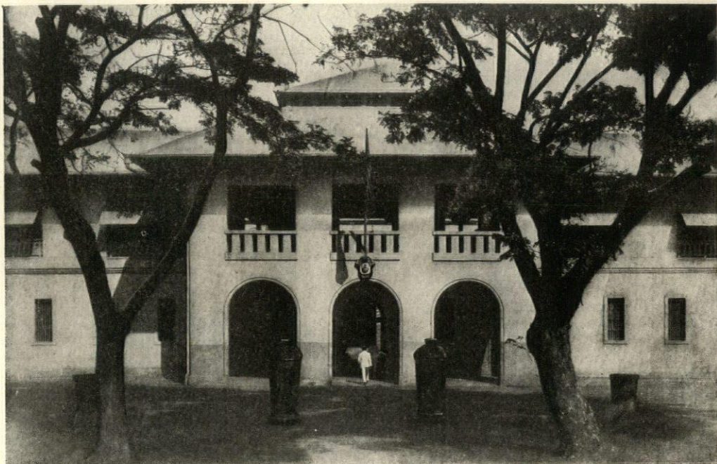
PROVINCIAL GOVERNMENT BUILDING, LAGASPI, ALBAY. 1907.
