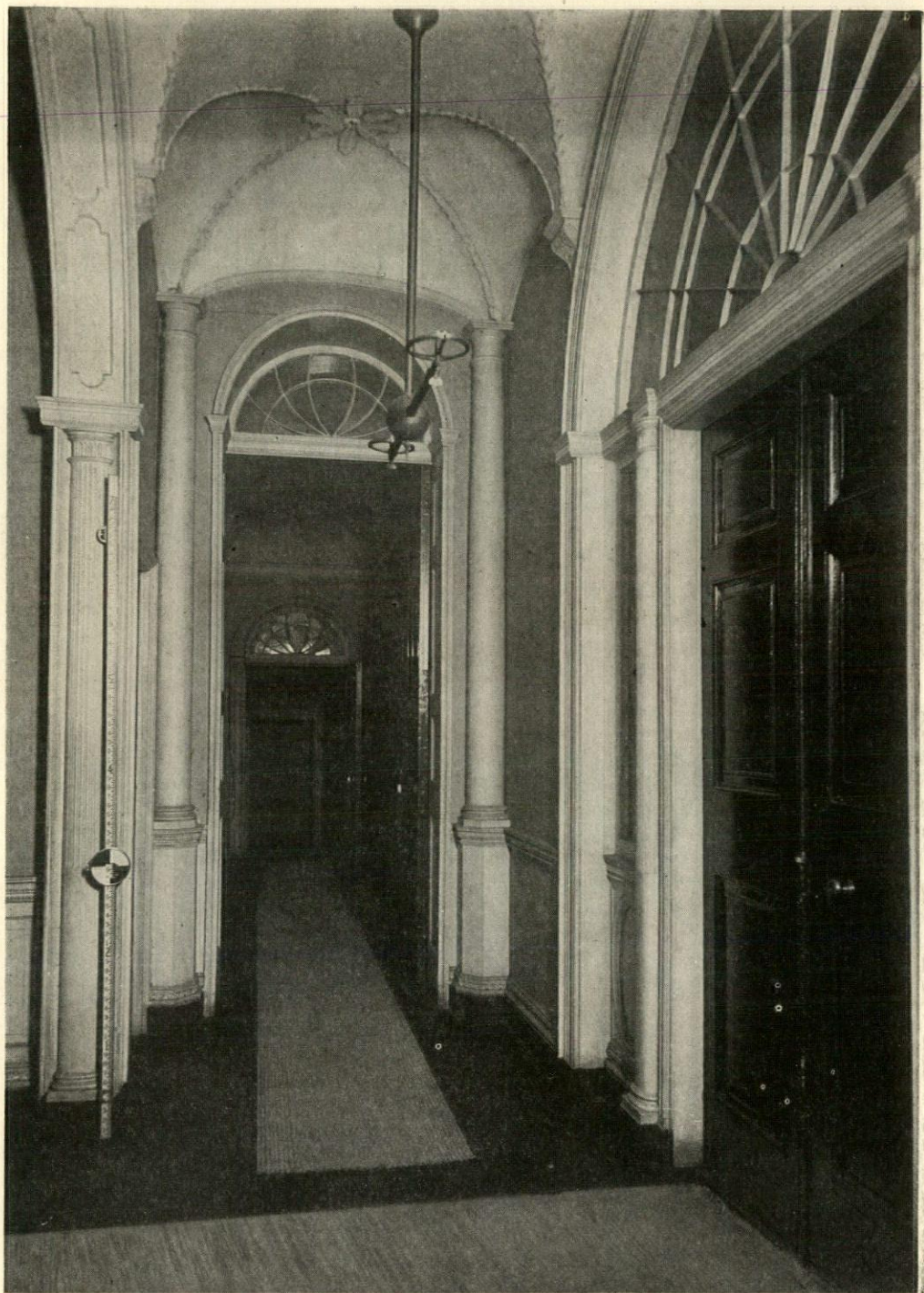
LOOKING DOWN LONGITUDINAL HALL OF HOUSE—HOMEWOOD, BALTIMORE, MD.
