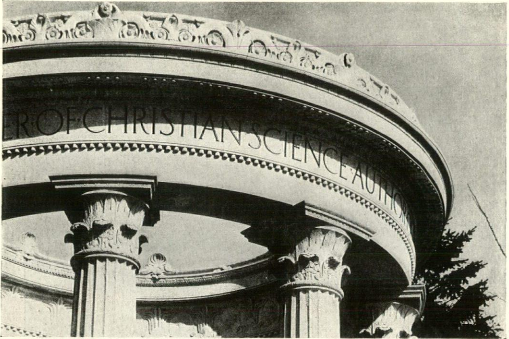
DETAIL OF ENTABLATURE—MARY BAKER EDDY MEMORIAL, MT. AUBURN CEMETERY, CAMBRIDGE, MASS. Egerton Swartwout, Architect.
