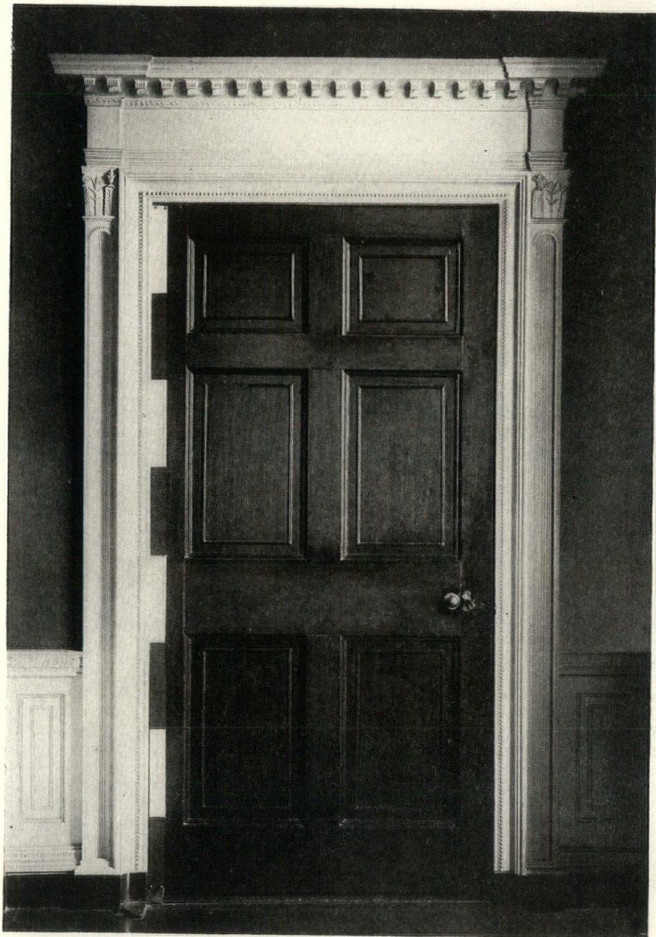
DOORWAY FROM LIVING ROOM TO SOUTH HALL—HOMEWOOD, BALTIMORE, MD.
