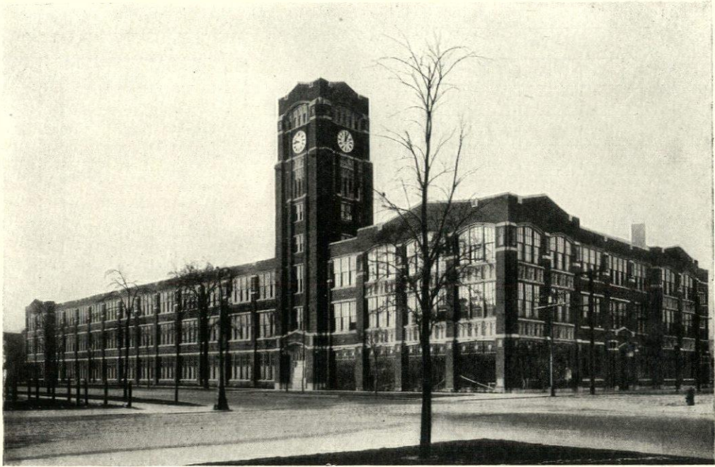
BUILDING FOR C. P. KIMBALL COMPANY, CHICAGO, ILLINOIS.
