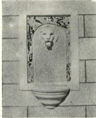
Surface Background Consists of Children's Beads Imbedded Flush With the Surface.
