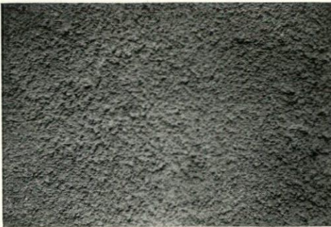
An Over-Coat Finish Called Sand-Sprayed. It Gives a Finer Texture Than Rough-Casting.
