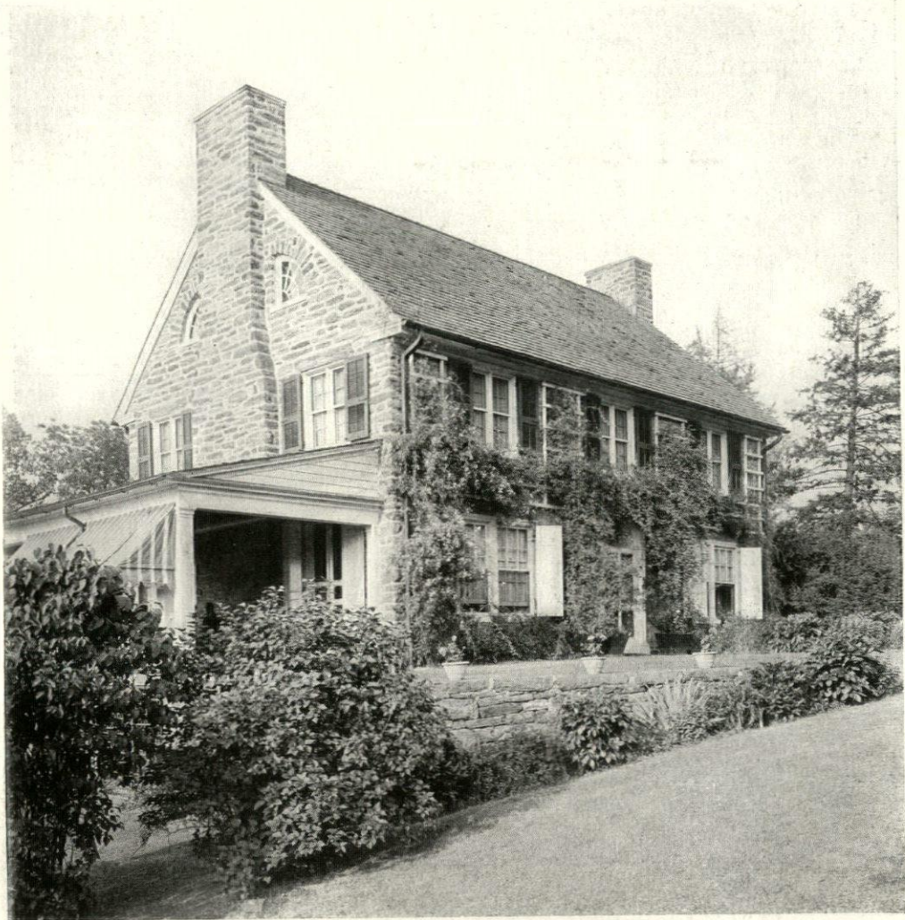
WEST FRONT—RESIDENCE OF MRS. FREDERICK PACKARD, CHESTNUT HILL, PHILADELPHIA, PA. WILLING & SIMS, ARCHITECTS.
