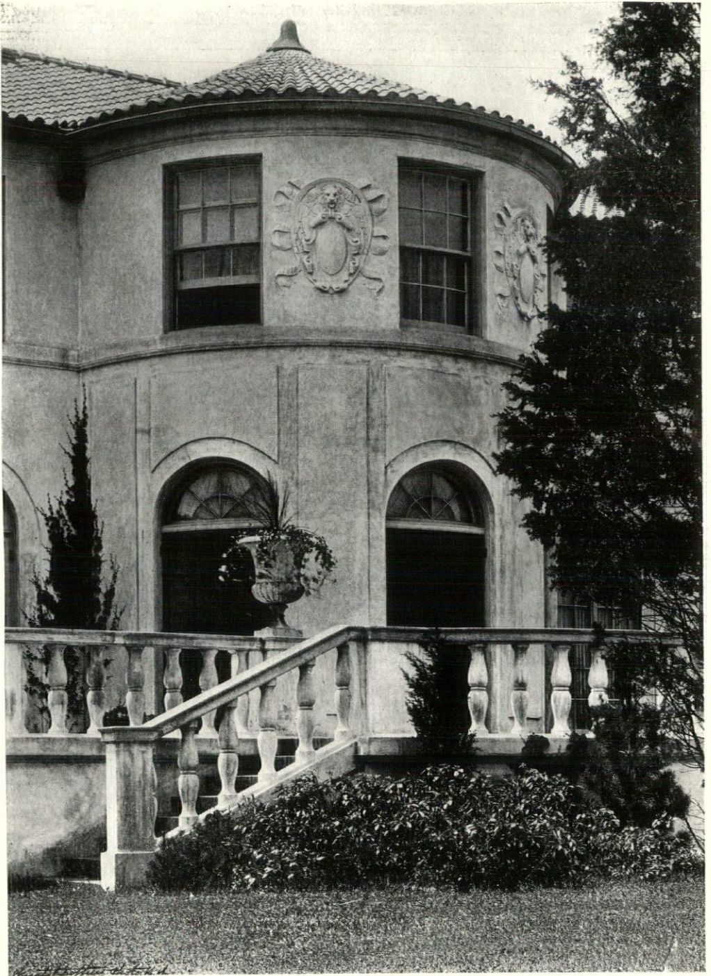
FIG. 1. DETAIL—RESIDENCE OF H. BELLAS HESS, ESQ., HUNTINGTON, L. I HOWELLS & STOKES, ARCHITECTS.
