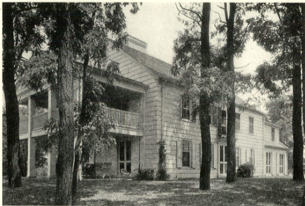
FIG. 39. WEST AND SOUTH FRONTS—RESIDENCE OF H. P. WHITNEY, ESQ., GLEN COVE, L. I. Charles Willing of Furness, Evans & Co., Architect.
