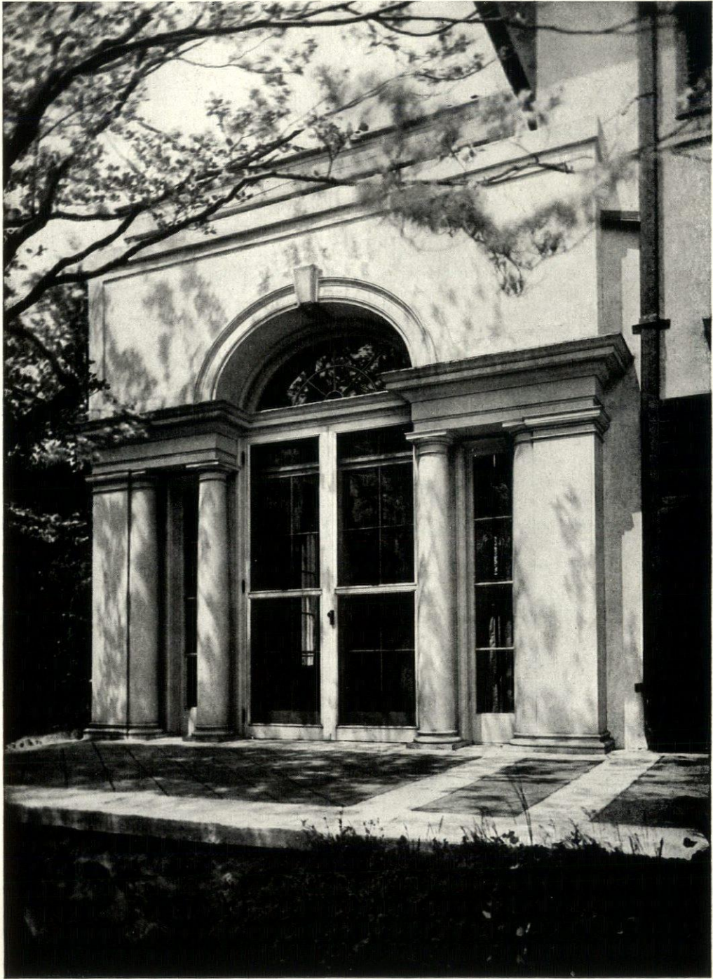
FIG. 3. SUN ROOM—RESIDENCE OF J. B. RICHARDSON LYETH, ESQ., FIELDSTON, NEW YORK CITY. DWIGHT JAMES BAUM, ARCHITECT
