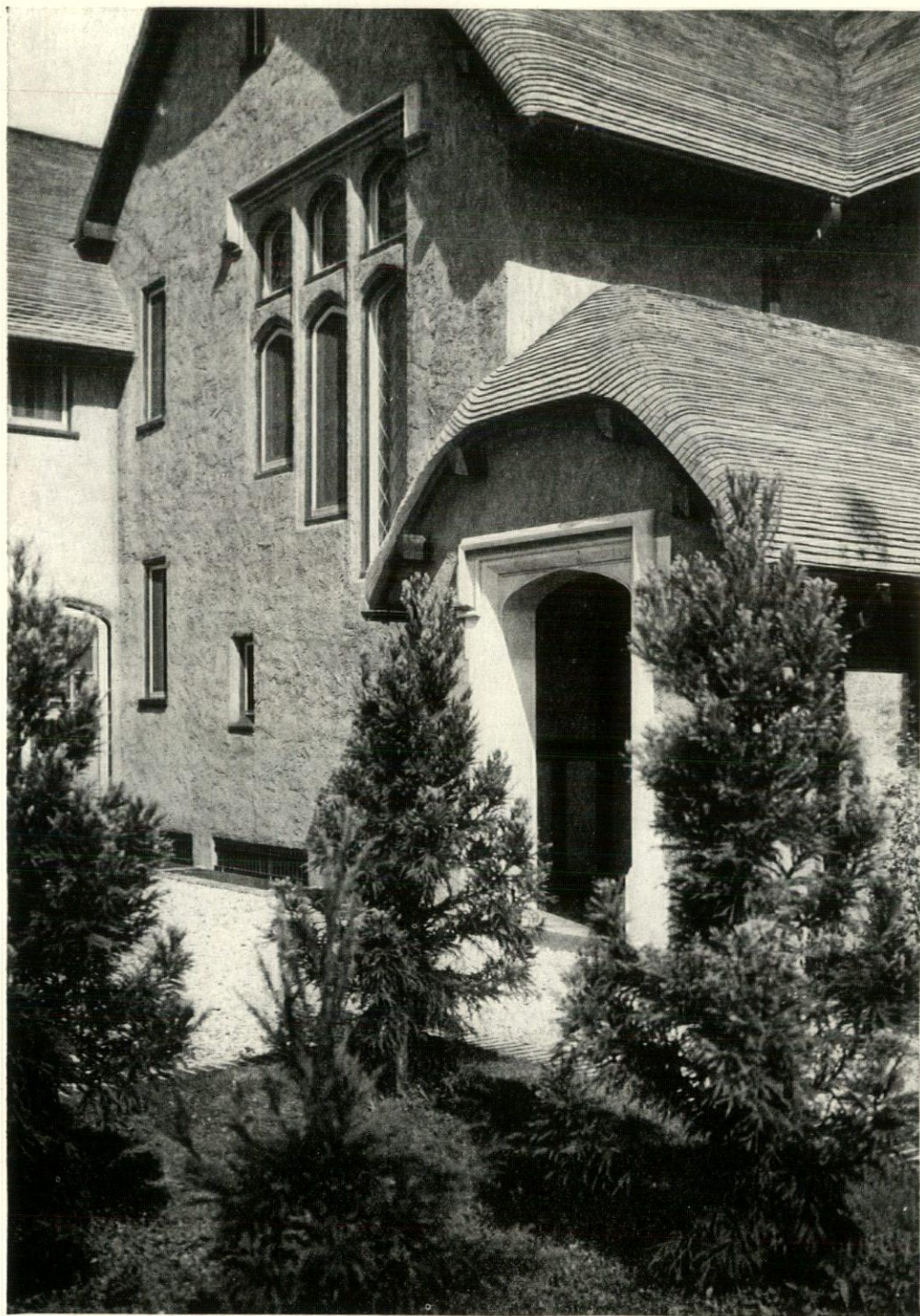
FIG. 110. RESIDENCE OF ROBERT APPLETON, ESQ., EAST HAMPTON, L. I. FRANK E. NEWMAN, ARCHITECT.
