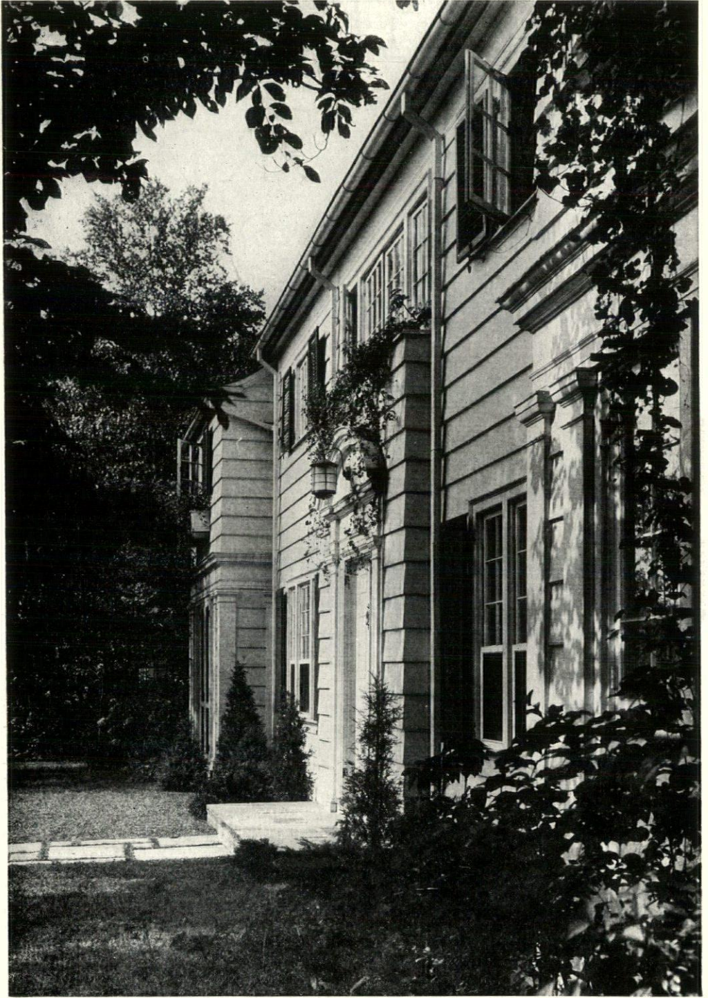
FIG. 2. DETAIL VIEW—RESIDENCE OF JOSEPH BUSH, ESQ., FIELDSTON, NEW YORK CITY. DWIGHT JAMES BAUM, ARCHITECT.
