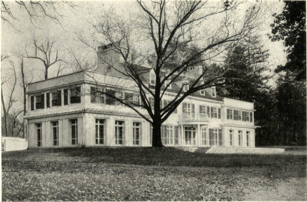
FIG. 61. RESIDENCE OF LEROY P. LEAS, ESQ., OVERBROOK, PHILADELPHIA, PA. Charles Barton Keen, Architect.
