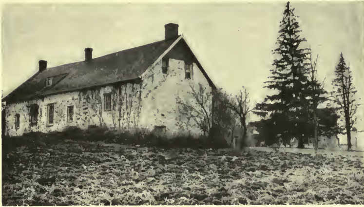
REAR VIEW OF HOUSE ON HIGHWAY NEAR MARBLETOWN, WITH EARLY DORMER. LIKE OTHER LONG HOUSES, USUALLY HAVING THREE CHIMNEYS, ITS KITCHEN DOOR IS ON THE FRONT.
