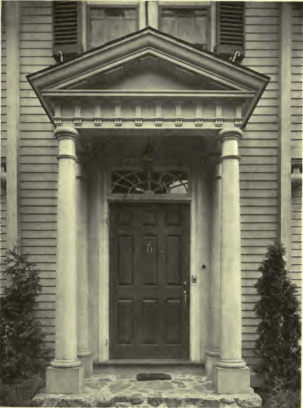
NORTH DOOR—RESIDENCE OF HERBERT S. DREW, ESQ., BELMONT, MASS. GRANDGENT & ELWELL, ARCHITECTS.
