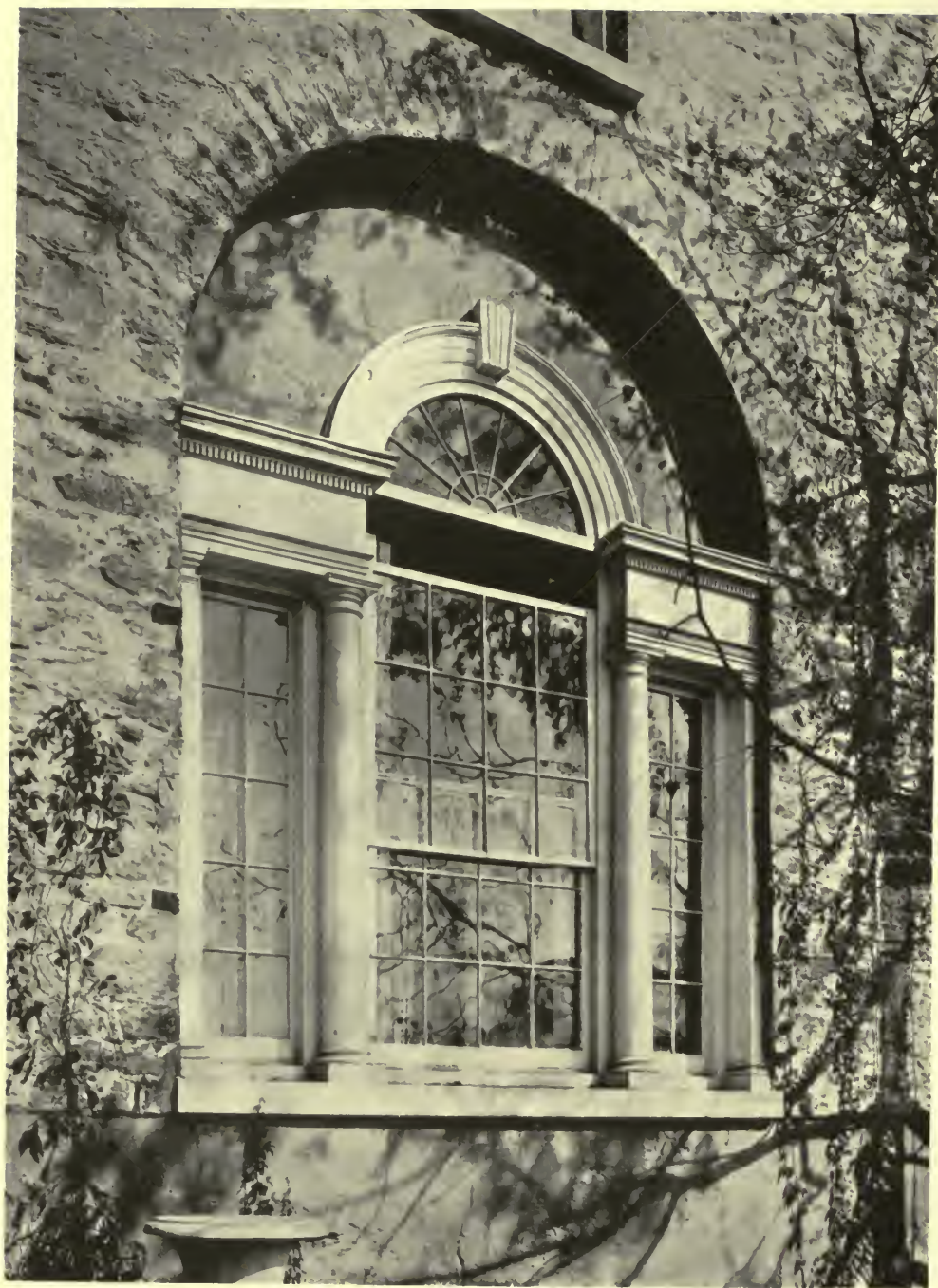
DETAIL OF PALLADIAN WINDOWS, "WOOD- LANDS," FAIRMOUNT PARK, PHILADELPHIA, 1770.
