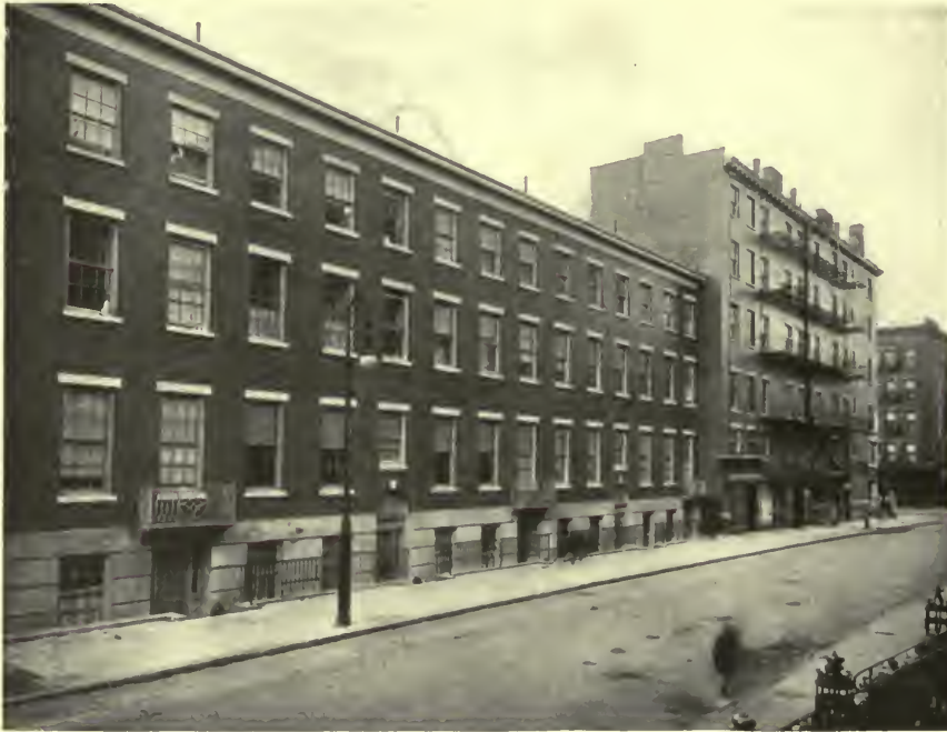
FIG. 8. DWELLINGS REMODELED INTO APARTMENTS AT 180 TO 188 SULLIVAN STREET, NEW YORK.
