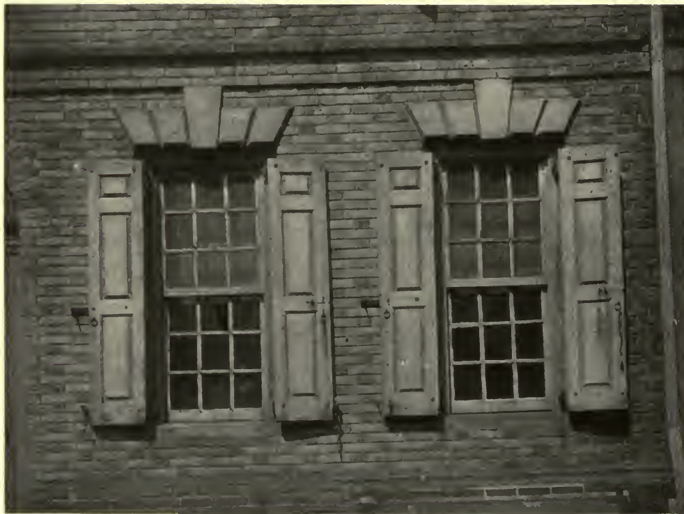
DETAIL OF WINDOWS, 514 SOUTH WATER STREET, PHILADELPHIA.
