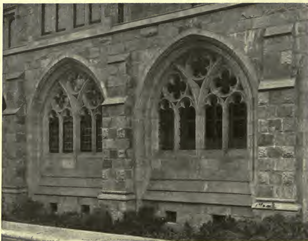
TRACERIED WINDOWS ABOVE MOAT-WALL IN ELM STREET— THE HARKNESS MEMORIAL QUADRANGLE AT YALE. James Gamble Rogers, Architect.
