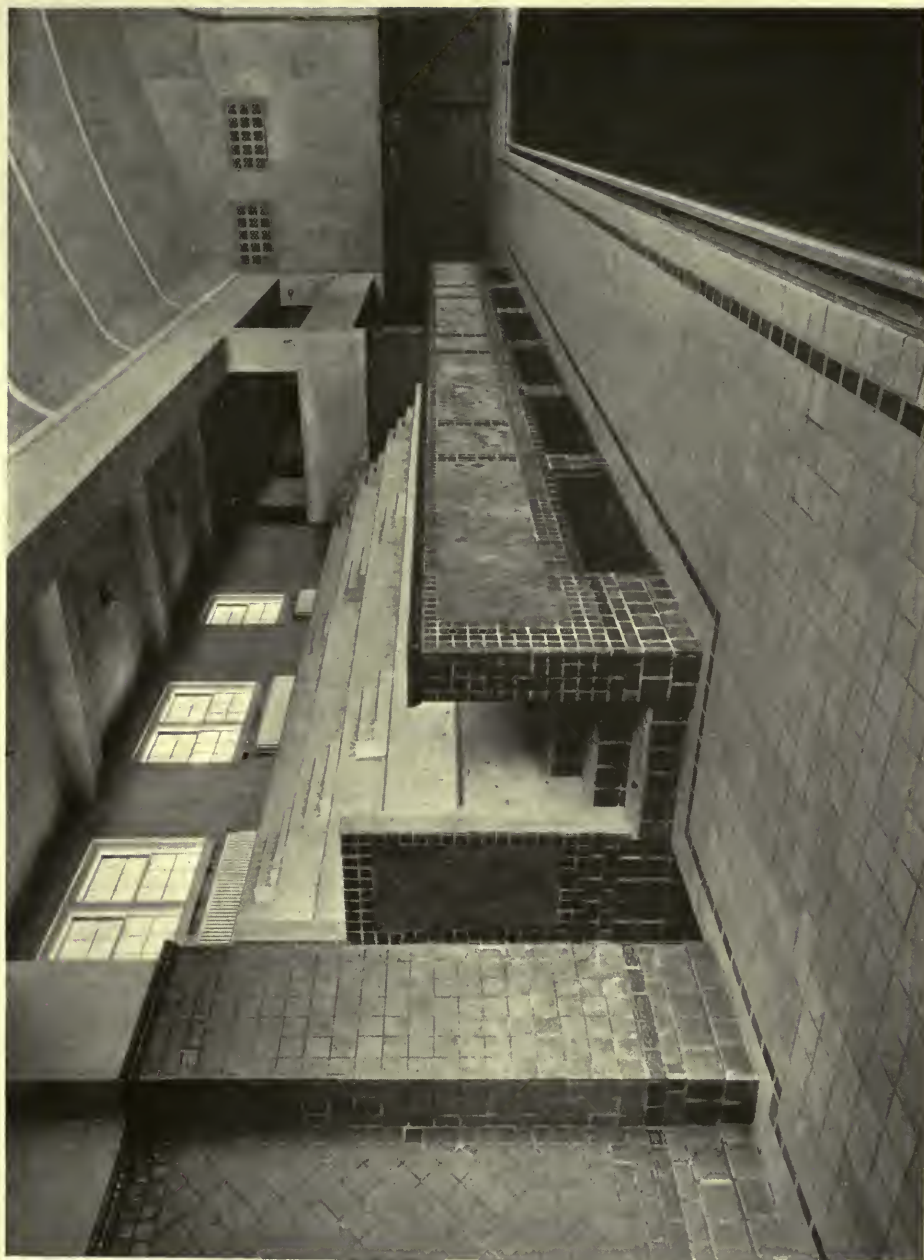
SPALDING SWIMMING POOL IN GYMNASIUM AT DART- MOUTH COLLEGE. RICH & MATHESIUS, ARCHITECTS.
