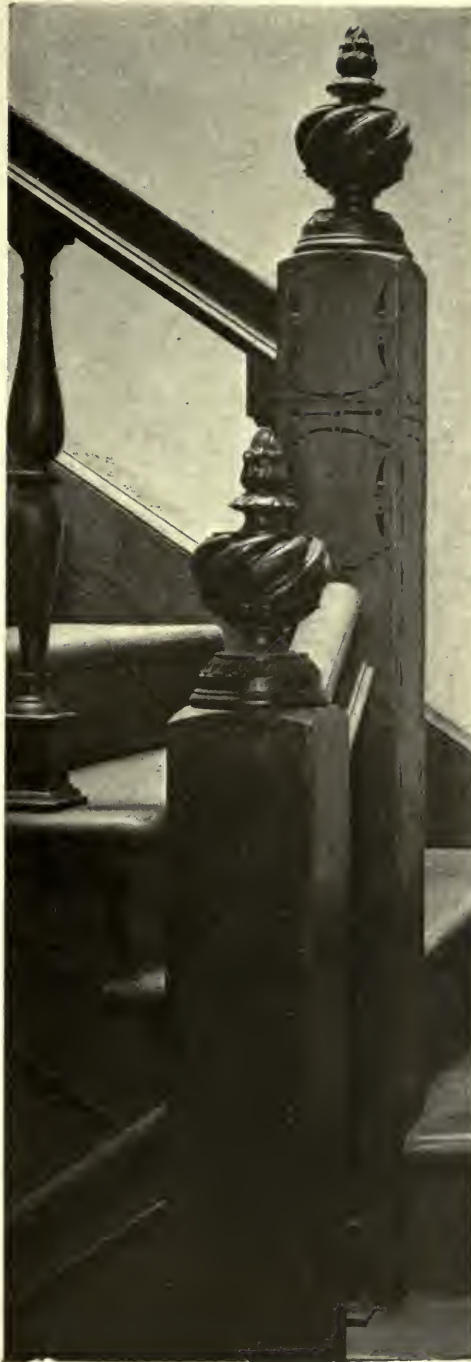
DETAIL OF STAIR NEWEL—RESIDENCE OF COLONEL MICHAEL FRIEDSAM, NEW YORK CITY. FREDERICK G. FROST, ARCHITECT.
