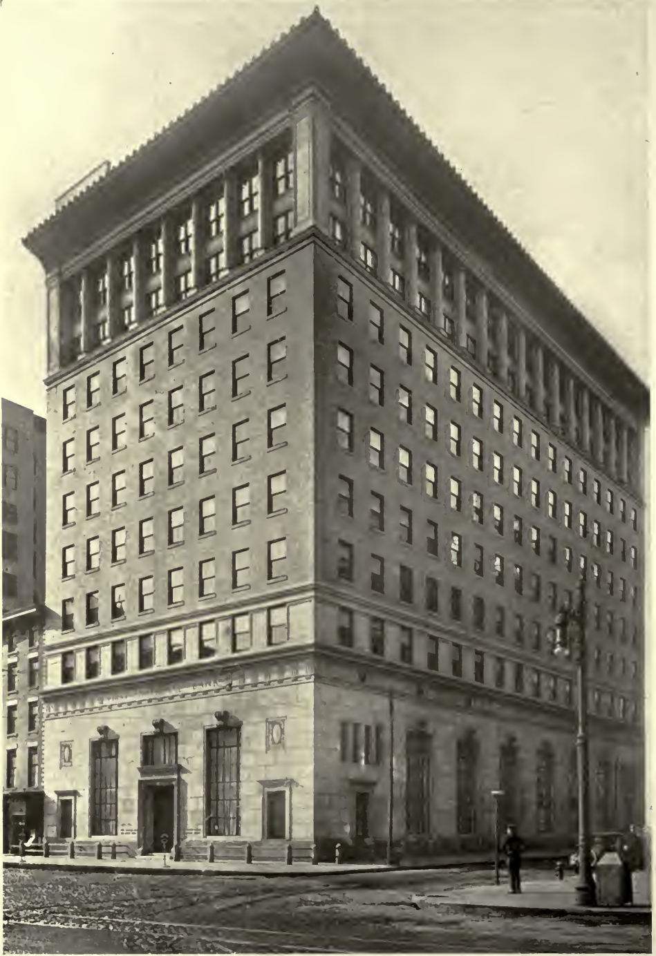
GENERAL VIEW—FIRST NATIONAL BANK, JERSEY CITY, N. J. ALFRED C. BOSSOM, ARCHITECT.
