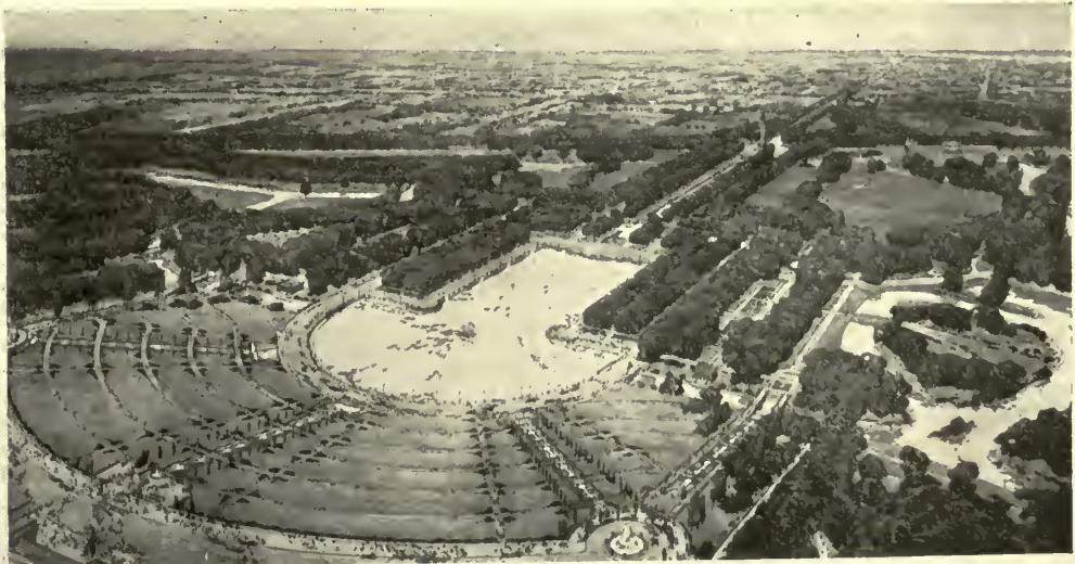
The Grand Basin of the World's Fair is retained in the Cass Gilbert plan for the restoration of Forest Park, St. Louis. The Festival Hall and Cascades which featured the Exposition have been removed and the amphitheatre regraded according to the new design.
