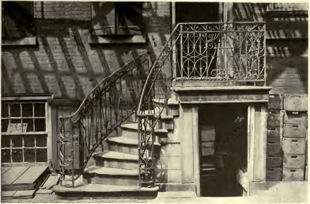
WROUGHT IRON PORCH AND STAIR RAIL, 272 SOUTH AMERICAN STREET, PHILADELPHIA.
