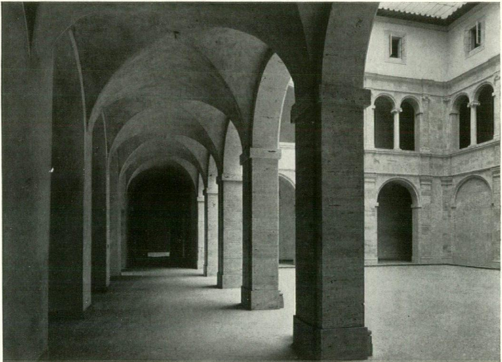
Corridor, First Floor
