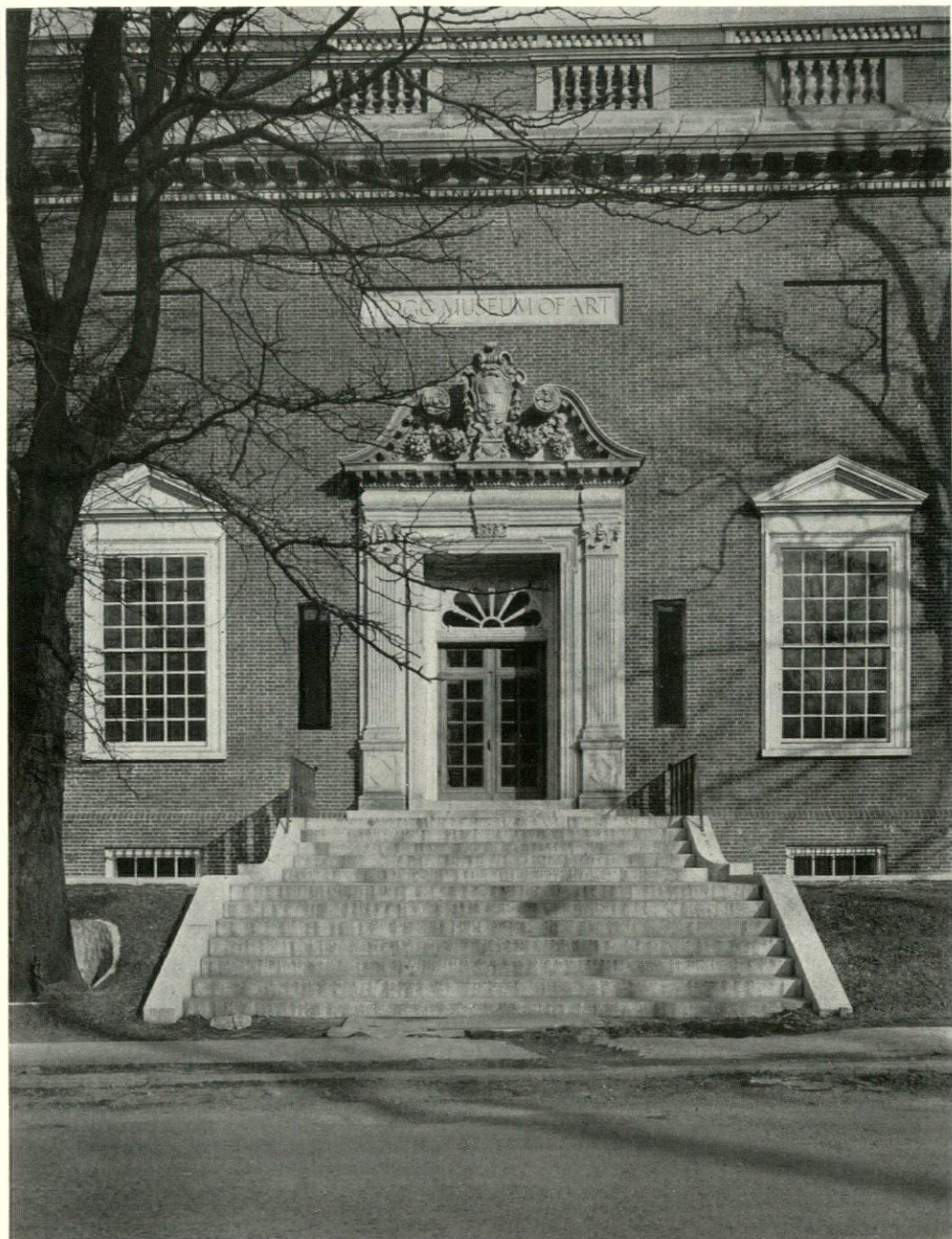
Detail of Main Entrance
