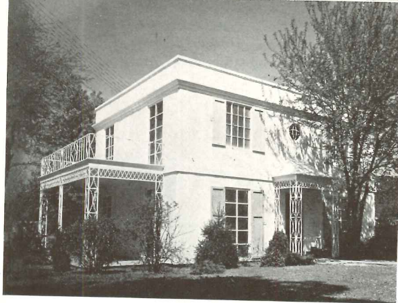
PREFABRICATION MOVES ON IN THE Midwest. The Cape Cod model (above) is all-steel arc-welded on the job, while the Regency was completely fabricated in the factory, trucked to the site. (For earlier Midwestern "truckable" houses see March 1937, page BT36.)
