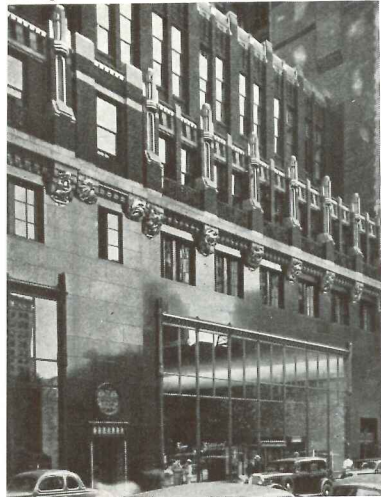
Addition shown on right half of photograph.
