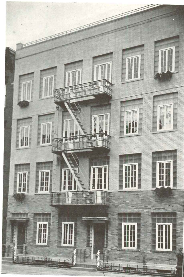
FOR BUILDING DESIGNERS PLAGUED with the limitations involved in remodeling old tenements on interior lots, Egmont Merseberger, Hoboken architect, has an idea: Enlarge glass areas in outside walls as much as structure will permit and set standard windows in the glass-block panel; replan interior
