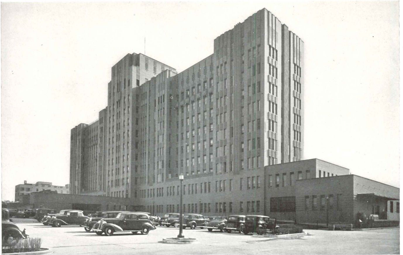
MAIN BUILDING, east elevation
