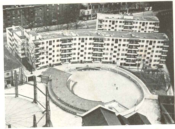
HOW TO USE GAS IN SLUM CLEARANCE. This recent project in London demonstrates not only the practicability of gas as a fuel but also of gas works as a site. 64 fireproof flats built around a nursery school on the site of a former gas tank.
