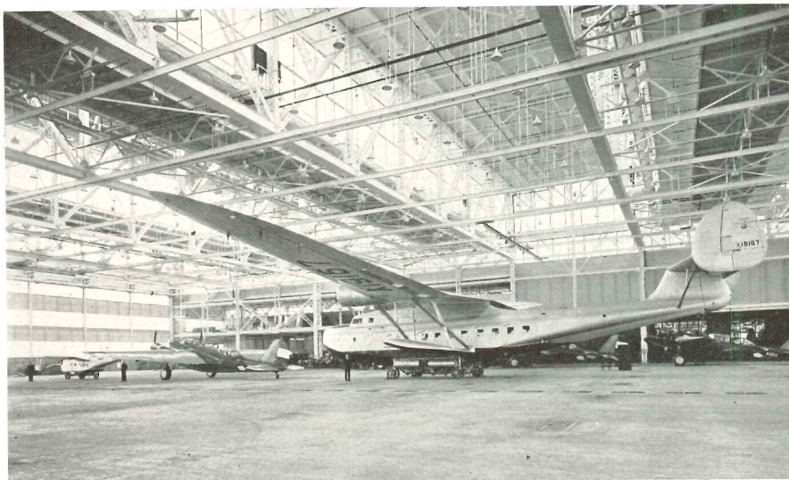
Upper: Facade of the Administration Building, with the Engineering Building in the background. Lower: Interior of the Assembly Building, 300 ft. wide, 450 ft. long, 40 ft. clear headroom throughout.
