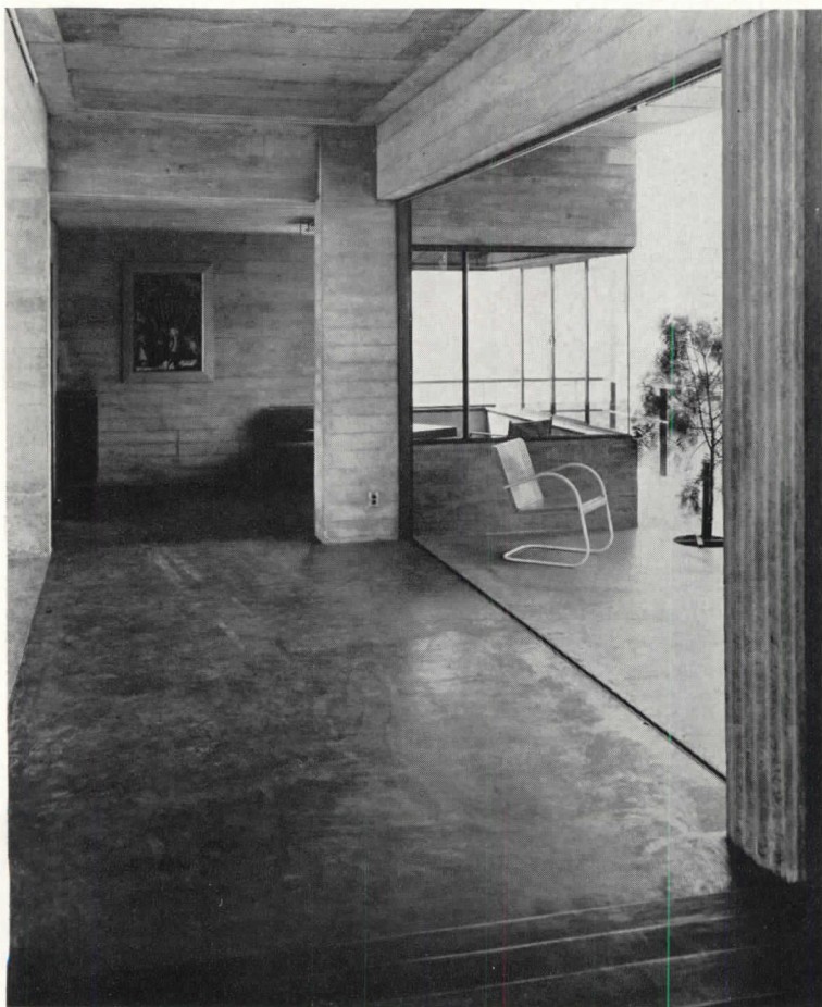
ABOVE: Living room, looking west. The elevated concrete hearth merges into three concrete steps crossing the width of the room. Hearth steps provide seating for a relatively large number of guests, without cluttering the room with too many chairs. LEFT: Dining room, seen from gallery; bay is cantilevered over canyon.
