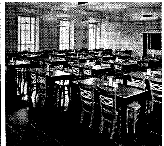
Lunch room is 39 ft. 6 in. by 53 ft.; contains 43 tables, 171 seats. Lighting is standard direct, diffused. Floor is rubber; base, slate; walls and ceilings, acoustic plaster.
