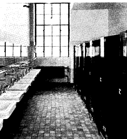
Washroom. These vary from 120 sq. ft. to 150 sq. ft. in size. Lighting is standard direct, diffused. Walls, floor, base, and dado are ceramic tile in shades of tan with white trim.
