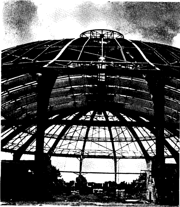
View of construction showing the rigid frames and the systems of purlins and bracing used.
