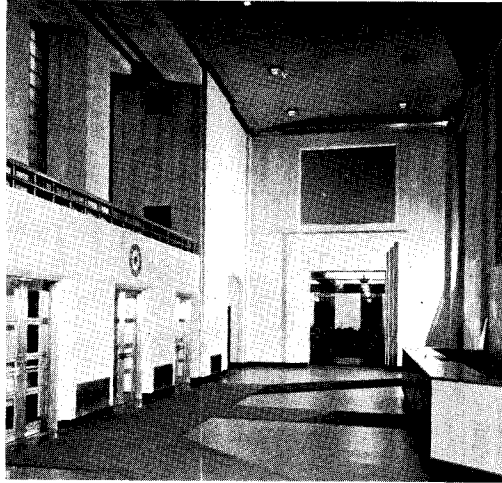
Main lobby is 22 by 72 ft., 27 ft. 6 in. high. Lighting is provided by 14 down-light projectors, 300 watts each. Floors are terrazzo; walls travertine with plaster panels for murals. Ceiling is painted medium blue.
