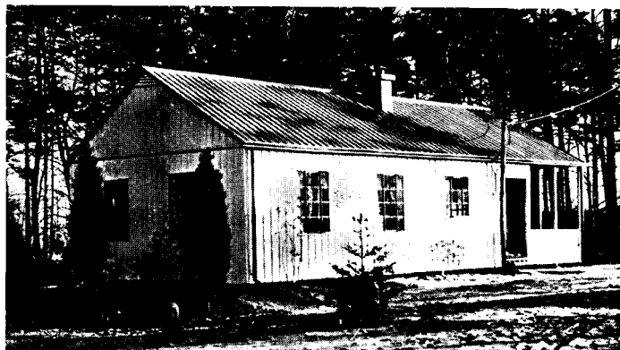
Fig. 16. One of a line of all-steel, shop-welded houses recently introduced in the South by United States Steel.
