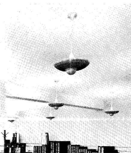
Totally indirect units in the Remington-Rand Building, Chicago, Ill.
