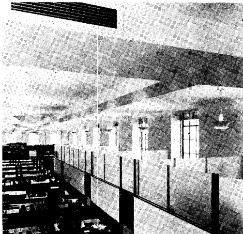
General office spaces have air-conditioning outlets at the faces of beams and are acoustically treated. Lighting is semi-indirect; colors having high reflectivities are used on walls and ceilings.
