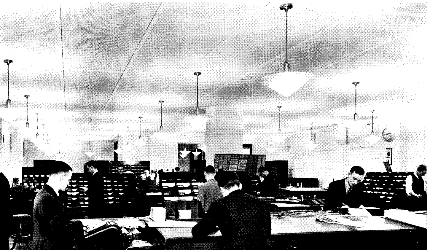
Semi-indirect fixtures 9 ft. on centers, bookkeeping department, Crocker First National Bank, San Francisco
