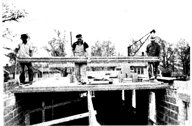
Fig. 7. Increasing variety of shapes in hollow tile yield possibility of prefabricated reinforced members. Typical unit employed (top) in prefabricated beams (bottom).
