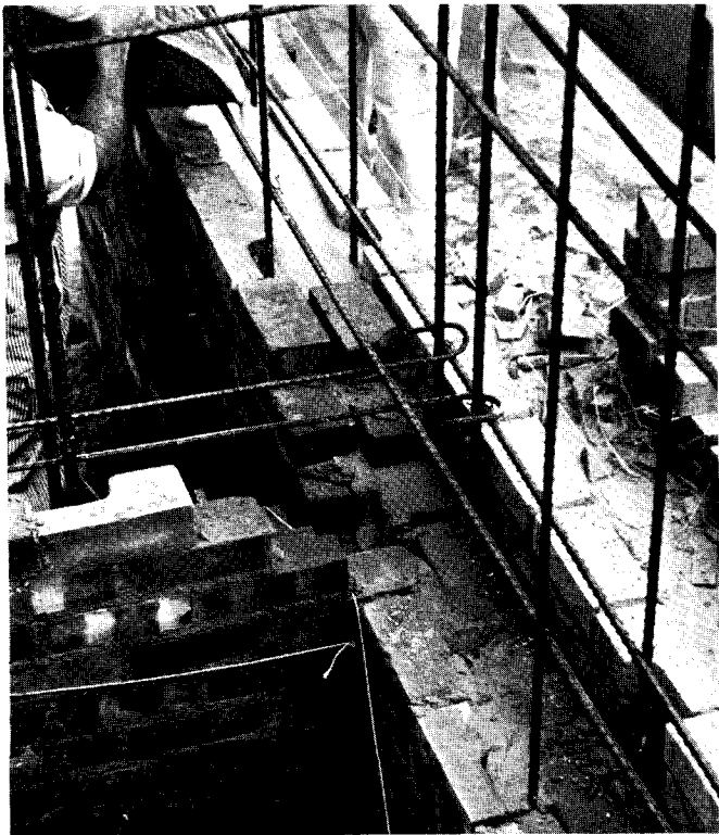
Fig. 6. Reinforced brick adds potentialities to the field of small-unit masonry construction, particularly valuable where unusual stresses necessitate structural flexibility.
