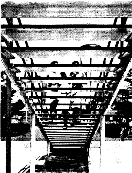
The Glass Center features treads of toughened glass on metal stringers.
