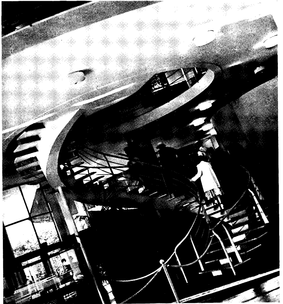
Ireland's reinforced concrete spiral stair has treads cantilevered from central spine.
