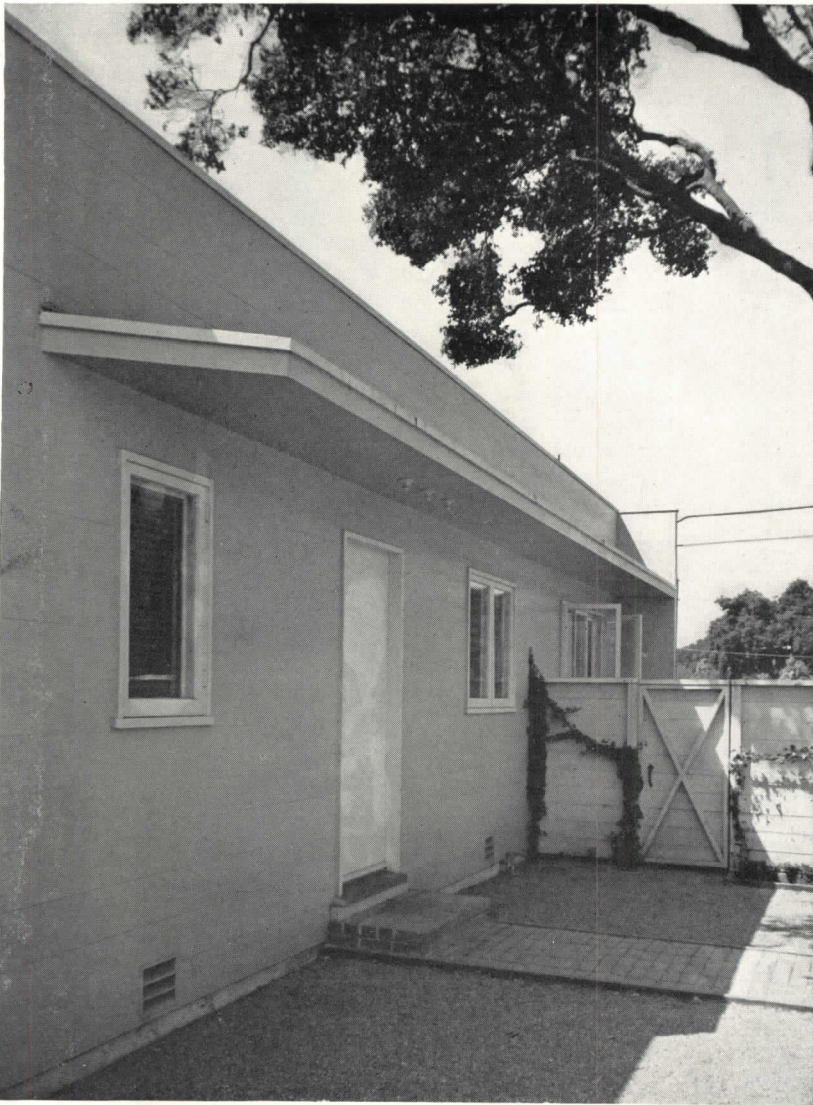
Fig. 16. Modern shiplap siding produces a flush exterior wall surface.
