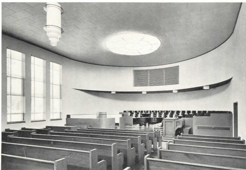
The chapel is semicircular at one end; this provides seating for the choir, each member of which has at least a side view of the speaker. For economy the organ is located in the slight overhang, with a grilled opening in the wall above the choir. Walls are of smooth plaster painted pale lime yellow.
