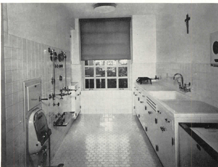
Utility room, St. Vincent's Maternity Hospital. Note bed-pan unit.
