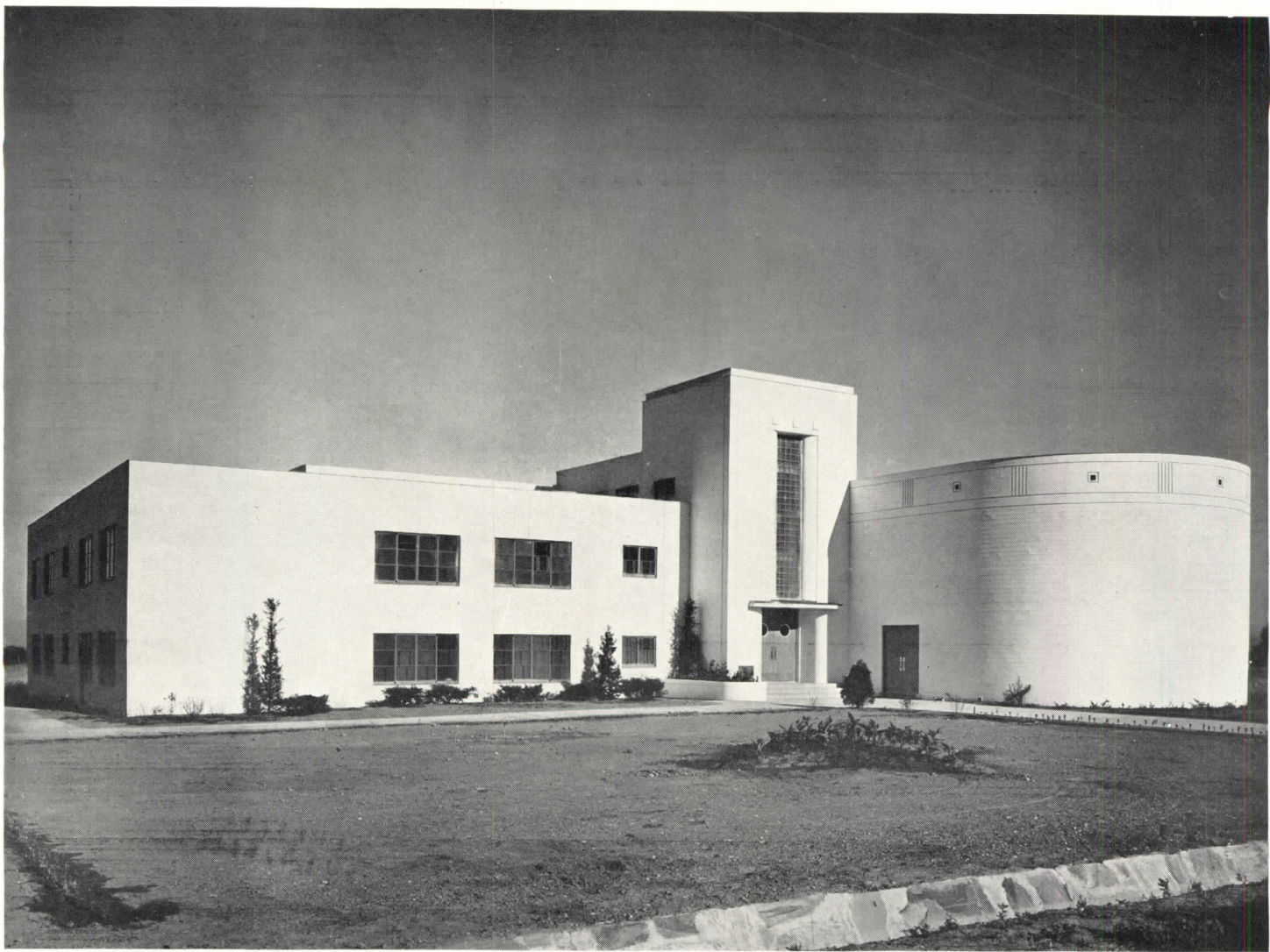
The marks of the form boards are left as a surface texture. All the sash are Soulé steel with felt weatherstrip.
