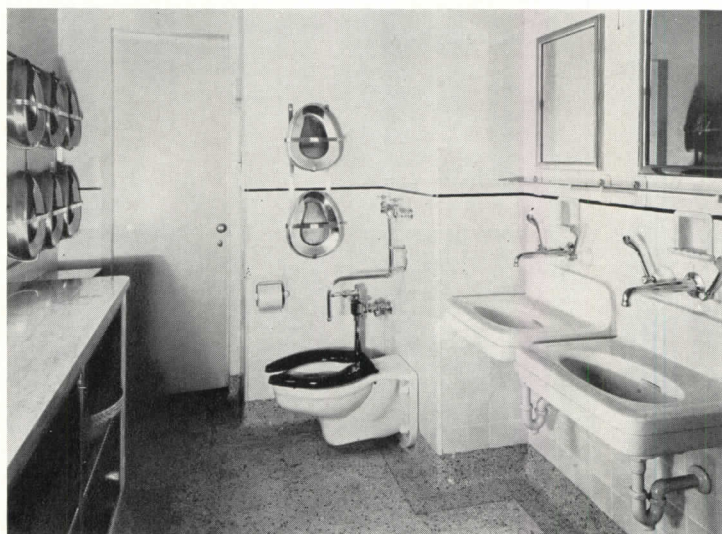
Service room for two four-bed wards, Chicago Lying In Hospital.
