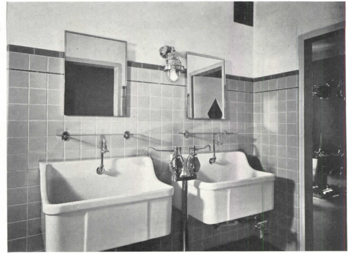
Scrub-up room, adjoining operating room at left; note knee-operated faucets and "explosion-proof" lights.
