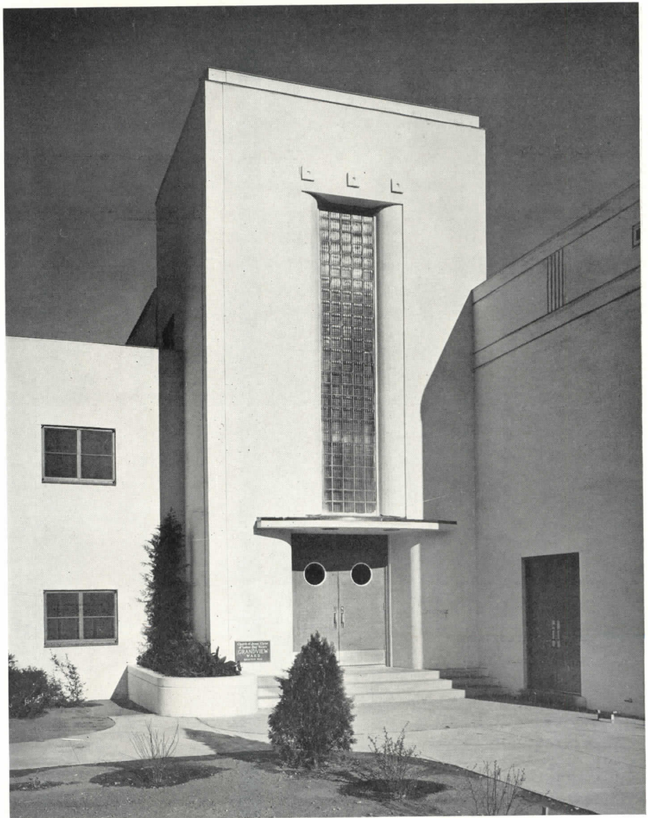
The two-story entrance tower dominates the design and separates the public and semi-public functions of the building. The vertical panel over the entrance is Insulux glass block.
