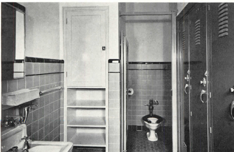
Service room, four-bed ward, St. John's Hospital, Springfield, Ill.; Henry R. Helmle, architect.
