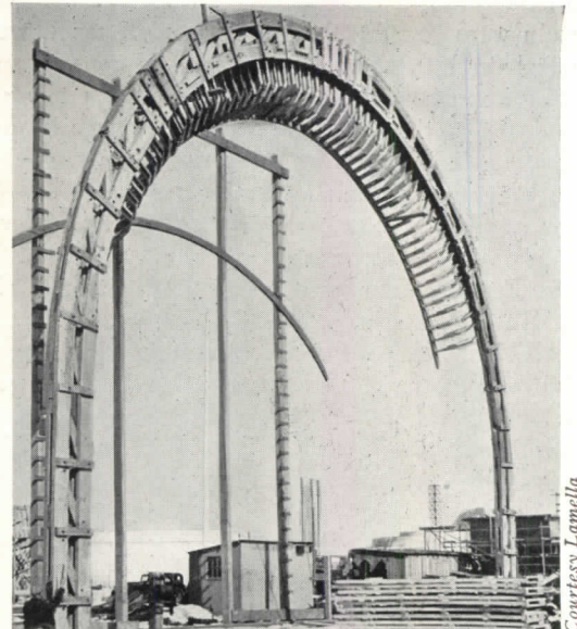
Fig. 6. A timber frame for a monumental arch.
