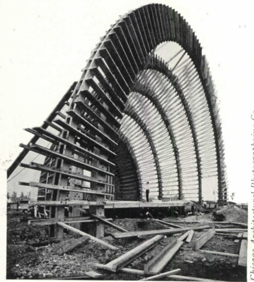
Fig. 2. As framing—all timber.
