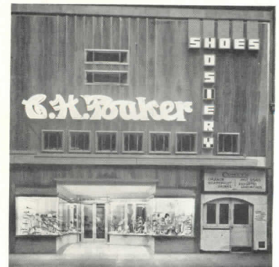
View of remodeled entrance
