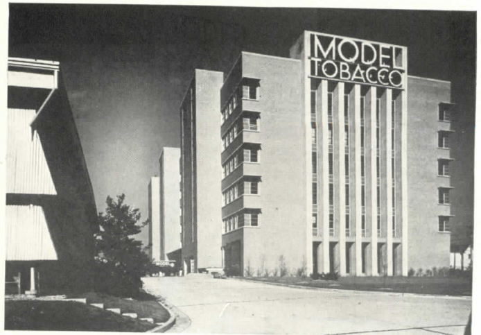
TRUCKING LANE (warehouse at left)
