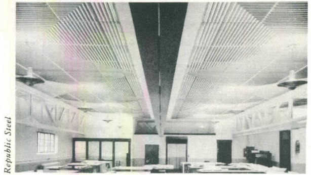
Fig. 10 WITH CORRUGATED METAL PANS of high reflectivity, the entire ceiling may act as a parabolic reflector, redirecting light downwards
