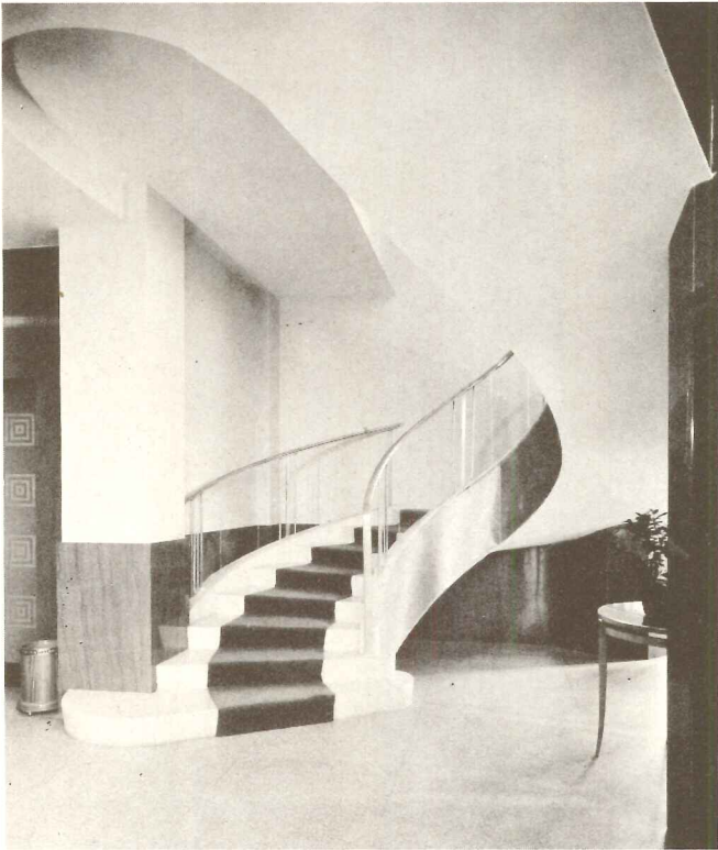
FREESTANDING STAIRS TO MEZZANINE have an etched clear plastic balustrade and aluminum handrail
