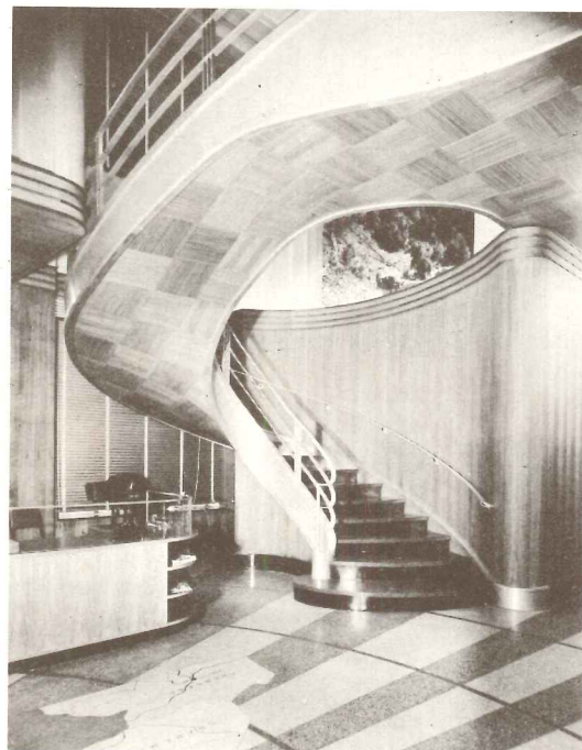
ALUMINUM HANDRAIL; wood veneer ceiling
