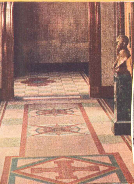
...razzo floor, made with Atlas White cement, in City Hall and Auditorium, Montgomery, Alabama. Architect, Frank W. Lockwood; General Contractor, Algernon Blair, both of Montgomery. Sub-contractor, Fornara Tile & Terrazzo Company, Atlanta.
