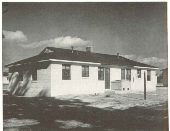
Rear service entrance of a typical house block
