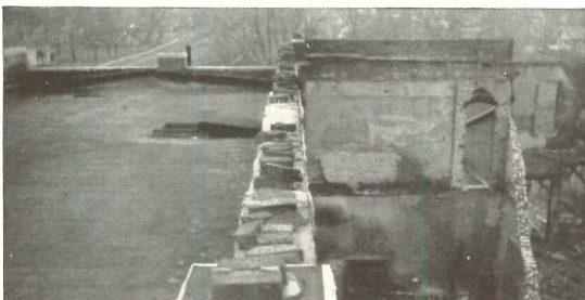
Although the low fire wall of the bank offered little protection, the flames were stopped by the J-M Asbestos Roof.
