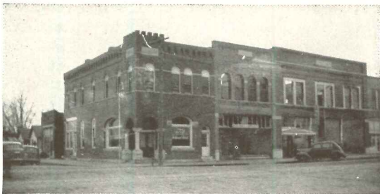
Starting in the building at the right, fire gutted the next two structures (see photo below), but a J-M Asbestos Roof saved the bank on the corner.
