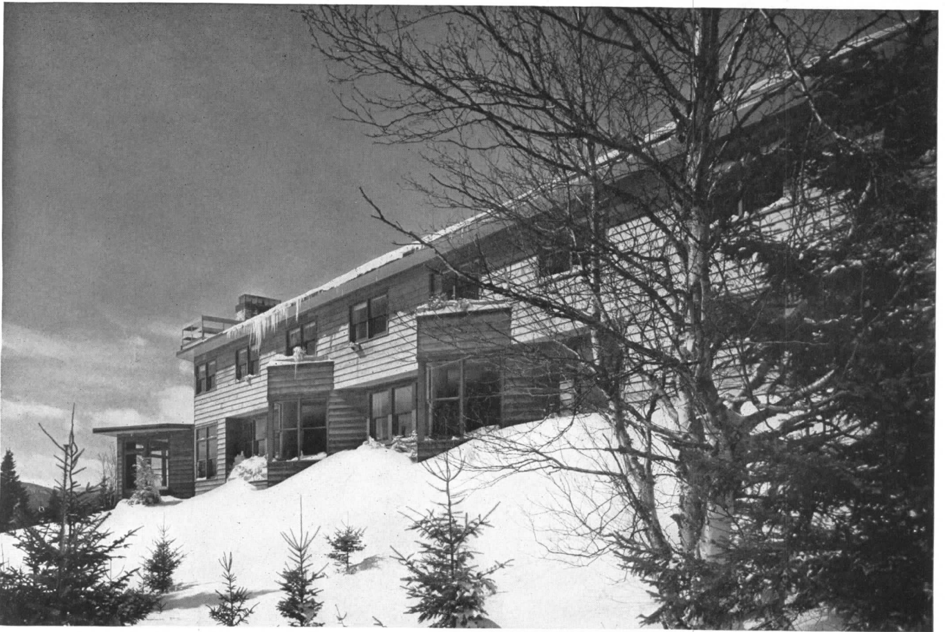
Form follows function in the design of the v-shaped alcoves which add interest to the facade and admit full sunlight to the classrooms
