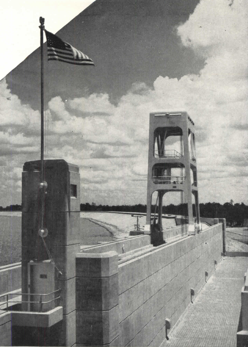
Top of powerhouse at Santee-Cooper power and navigation project 50 miles north of Charleston, S. C.
