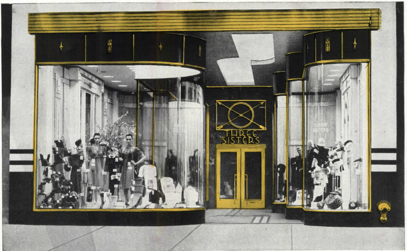
Three Sisters Store, Chicago, Illinois. Anaconda Architectural Bronze installed by J. S. Heath Company, Mitchell Corporation, North Chicago, Ill., successor.
