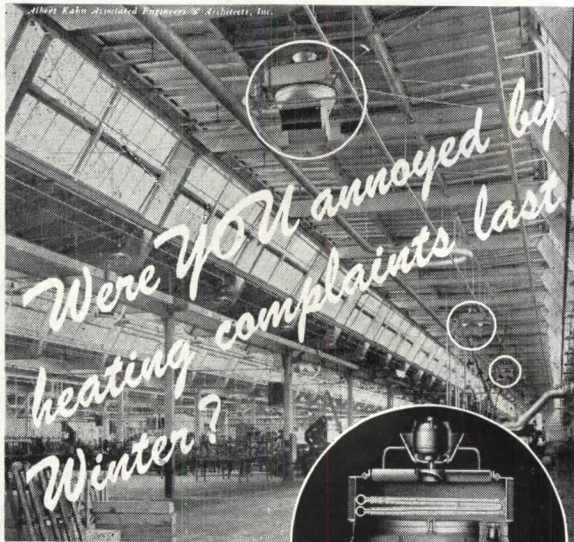
(Above) Installation of 63 Wing Revolving Unit Heaters in Plant of Automotive Appliance Manufacturer
