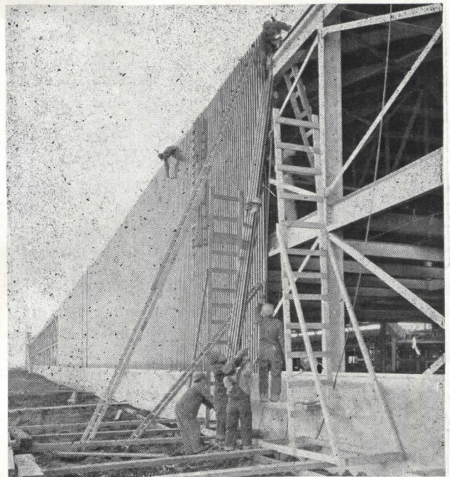
Robertson cellular steel wall panels, enclosing North American Aviation plant, Dallas. Gordon Turnbull, architect
