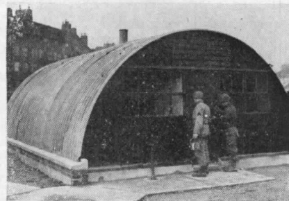
GI finishing touches and GI approval
