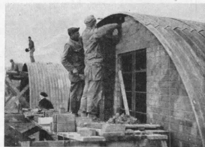
Two GI's bricking in the end of a hut
