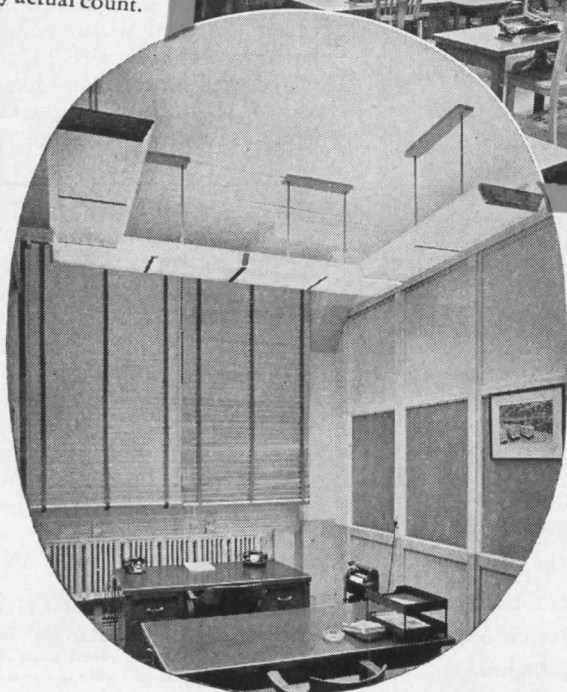
Private Office—a difficult lighting problem solved by coordinating desk and luminaire layouts. Maximum seeing comfort is provided with 85 footcandles on the worktable after 1000 hours burning.
