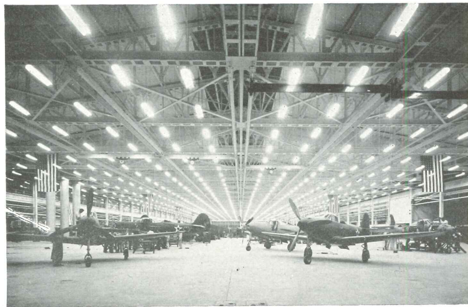
4. In a large interior, with high ceilings, the fixtures should be hung as high as possible. (Bell Aircraft plant, designed by the Austin Company)
