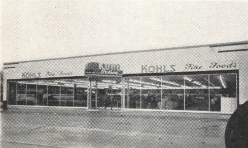
Thermopane in Visual Front of Kohl's Fine Foods, Milwaukee, Wisconsin. Architect: Walter F. Liebert, Milwaukee.
