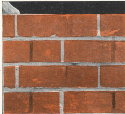
This encourages the bricklayer to fill the head joints, since proper tooling cannot be done if mortar is lacking.
