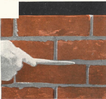
As an alternate for backplastering, the joints on the back of the face brick may be tooled to give a concave finish.
