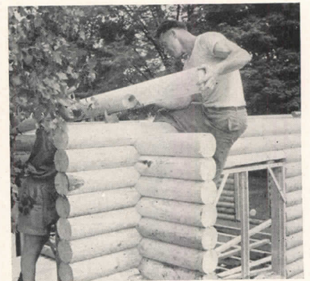
Ready-made logs aid rapid construction
