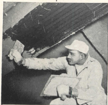
PUT ON THE PLASTER! Note the Monel Tie Wires holding this steel screening in place. Monel resists corrosion by alkalis and salts in plaster, lime and other building materials.
