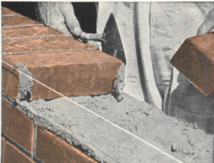
When mortar is spotted on both corners of the header brick,
