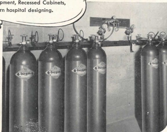
CENTRAL OXYGEN PIPING SYSTEM
