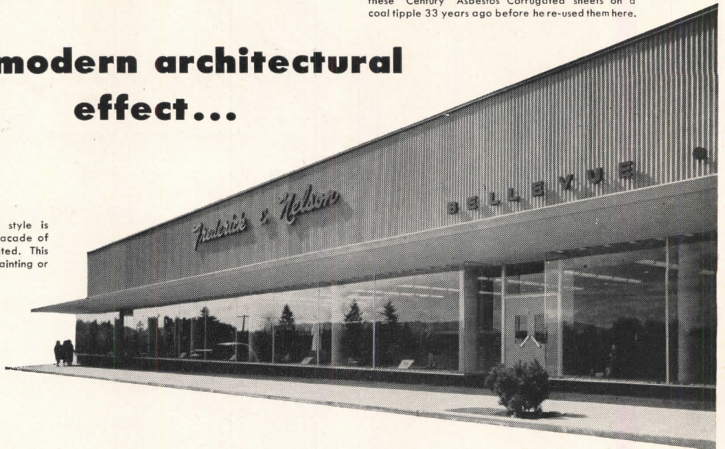
The "new" roof on this industrial building is actually more than 3 decades old! A coal operator installed these "Century" Asbestos Corrugated sheets on a coal tippie 33 years ago before he re-used them here.
