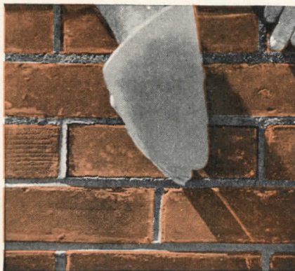
Realignment of a brick should not be attempted after a higher or following course has been laid. When a brick is hammered back into line, the bond between the brick and mortar is broken. Cracks due to such realignment are frequently found at the corners of the wall.
