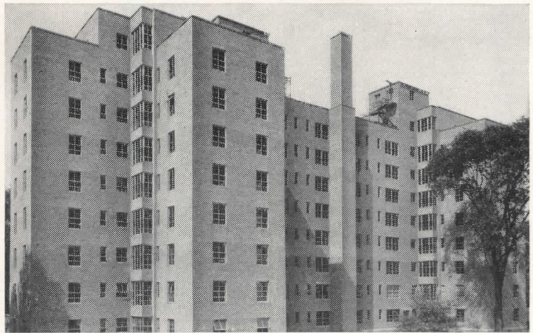
WHERE QUALITY ALONE COUNTS — TUDOR PLAZA APARTMENTS. For this ultra-modern cooperative apartment building in Buffalo, Gold Bond Partition Systems met all requirements.
