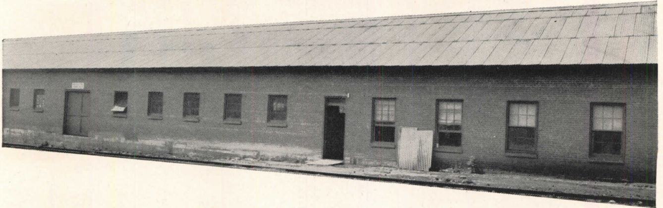
The "new" roof on this industrial building is actually more than 3 decades old! A coal operator installed these "Century" Asbestos Corrugated sheets on a coal tippie 33 years ago before he re-used them here.
