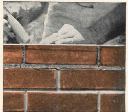
its position should never thereafter be changed. Shifting the brick breaks the bond between the brick and the mortar, and causes cracks in the wall.
