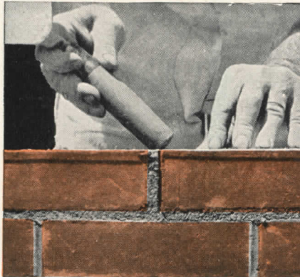
its position should never thereafter be changed. Shifting the brick breaks the bond between the brick and the mortar, and causes cracks in the wall.
