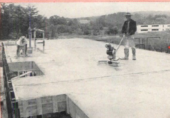
3 Two-inch concrete floor has been poured and finishing operations are under way.
