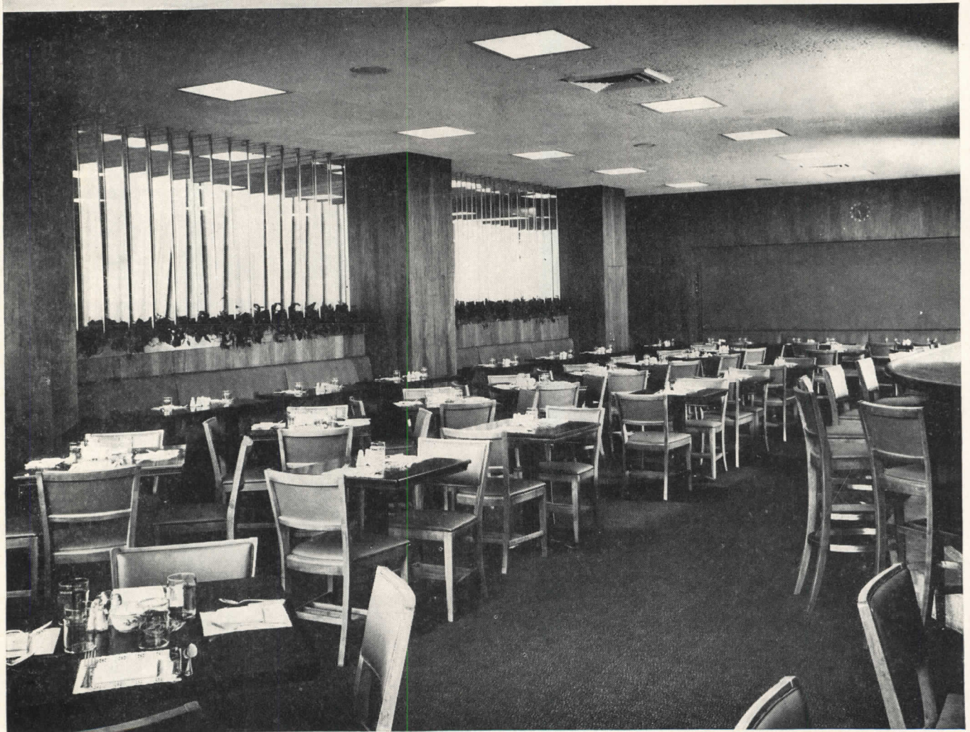
Versatile Agitair Type R's in Schrafft's Rockefeller Center, New York blend perfectly with surroundings, yet supply 100% air distribution. Other Schrafft's Located in New York, Boston, Syracuse, Philadelphia and Newark.
