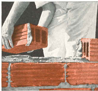
Method 2. A full head joint should be thrown onto one edge of the tile in place and also onto the opposite edge of the tile to be placed.
