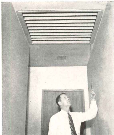
Pull on chain opens shutter and starts fan
