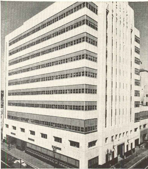
The Mirror Building, Los Angeles
