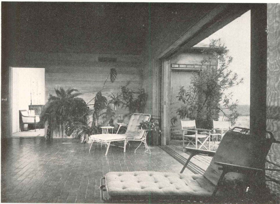
Rolling louvered shutters in combination with the glass doors permit the gallery to be breezy even in inclement weather
