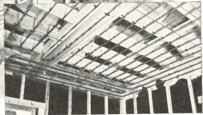
Ceiling installation of Radiant Panels
