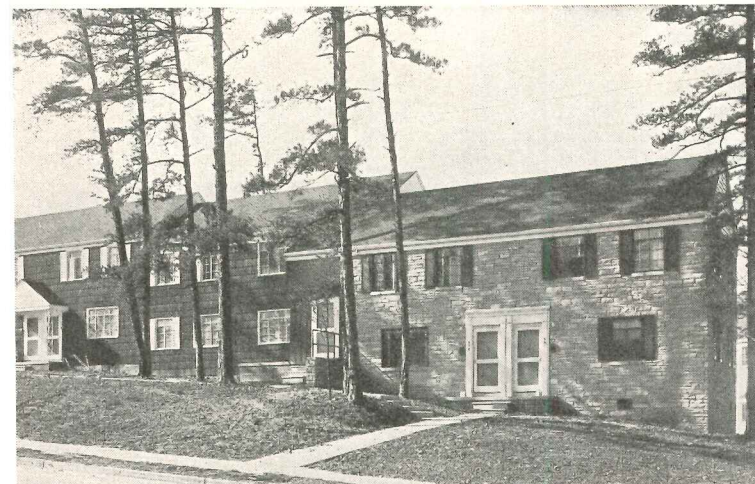
Exteriors of these garden apartment buildings are varied stone, brick or shingles. Two types of exteriors are shown above.
