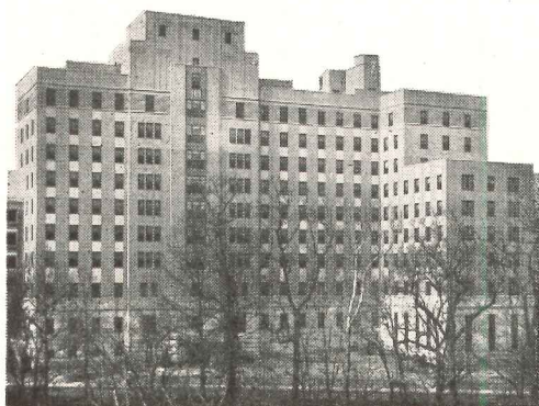
DELAWARE HOSPITAL , Wilmington, Del. Massena & Du Pont, Inc., Architects Turner Construction Co., General Contractor
