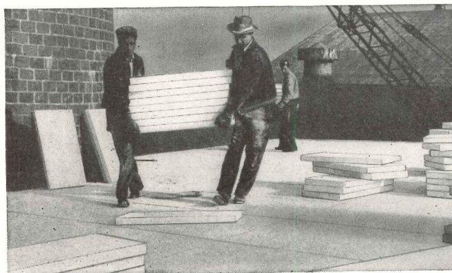
Two men here carry 8 Kaylo Roof Tiles while walking on roof deck already laid.
