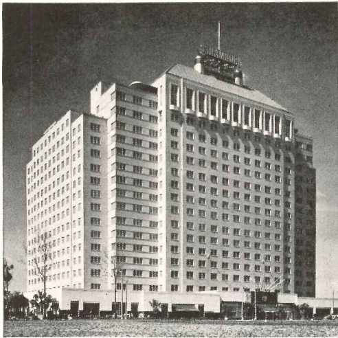
Construction Manager: STONE & WEBSTER ENG. CORP. Architects-Engineers: WYATT C. HEDRICK Air Conditioning Contractors: ASSOCIATED MECHANICAL CONTRACTORS
