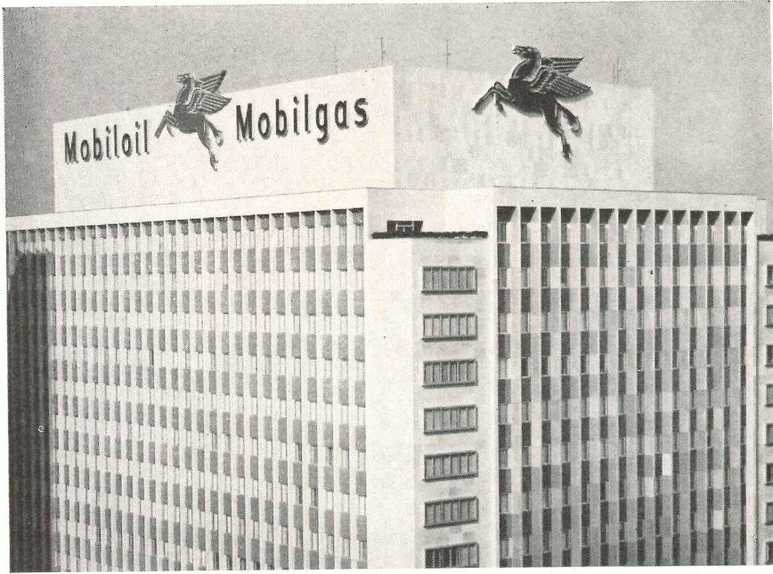
GENERAL PETROLEUM BUILDING, LOS ANGELES, CALIFORNIA
