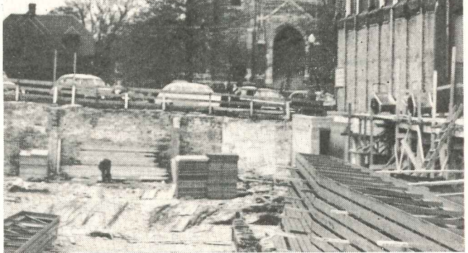
Truscon "Clerespan" Joists were used to obtain large unobstructed areas in the Star Market, Newtonville, Mass.
