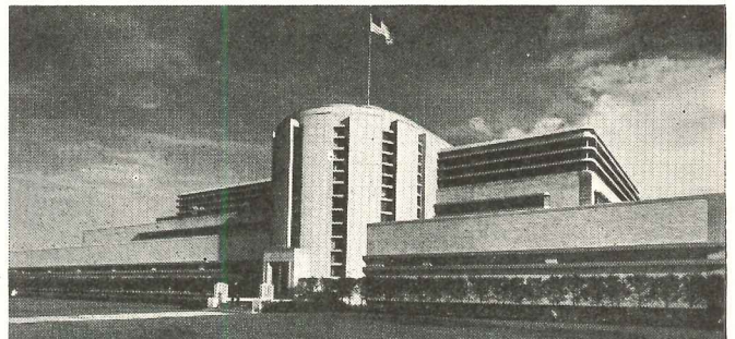
Modern, completely air conditioned plant, built by Geo. A. Fuller Co. for G. D. Searle & Co., Chicago, manufacturers of ethical pharmaceuticals.
