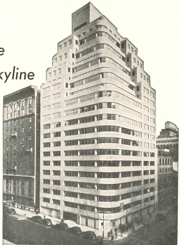
This recently completed office building in New York City contains 600 Weldwood Fire Doors. Uris Brothers Construction Co. built it. Designing architects were Emery Roth & Son. One of many major installations using Weldwood Fire Doors.
