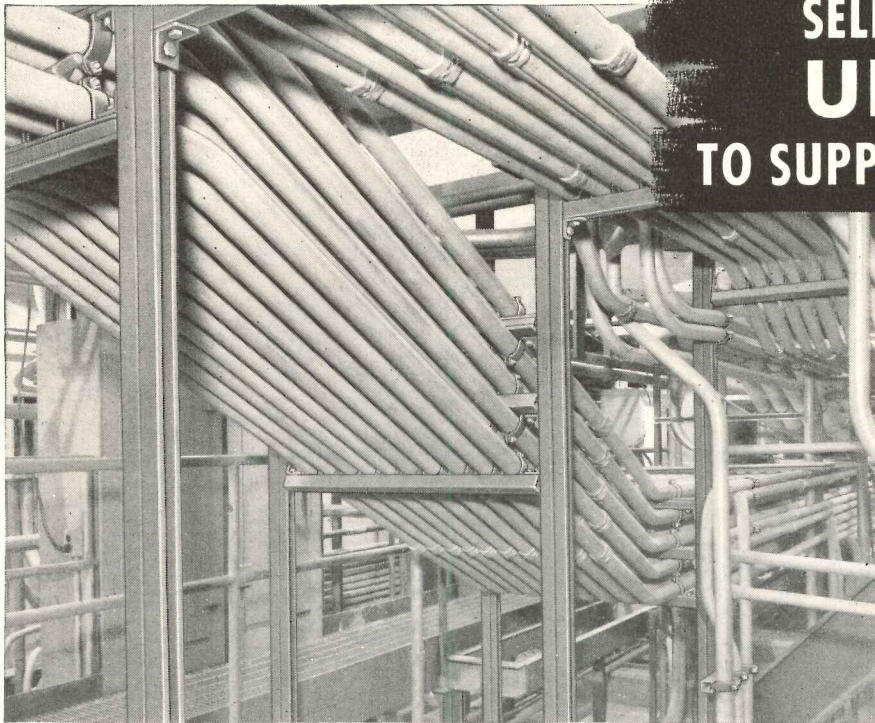
Heavy rows of conduit are quickly installed and easily supported with completely adjustable Unistrut channel, fittings and clamps. Note examples of combination racking where conduit is clamped above and below to channels mounted back to back.
