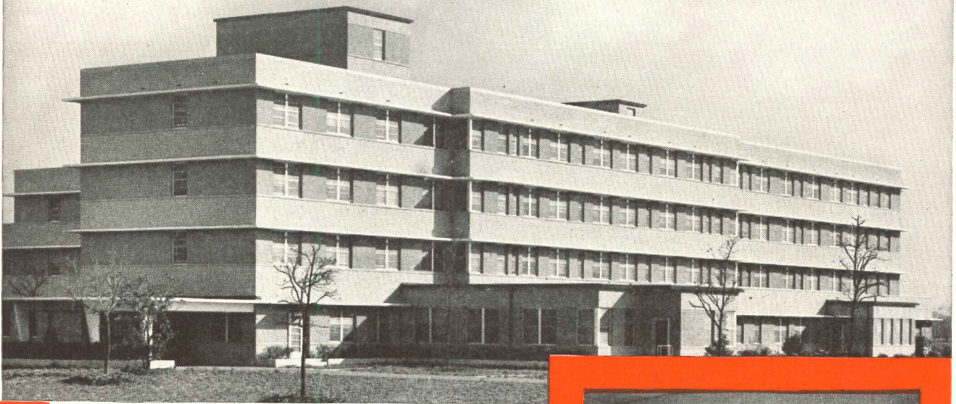
Baptist Hospital, Beaumont, Texas. Architect: Wyatt C. Hedrich, Dallas, Texas. Contractor: R. P. Farnsworth Co., Inc., Houston.
