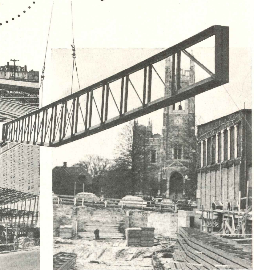
Truscon "Clerespan" Joists used in Adolphus Garage, Dallas, Texas.
