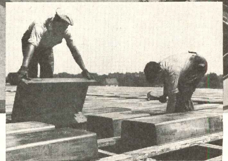
Labor of placing and removing steel-forms by skilled Ceko workmen is ordinarily included with the rental charge.
