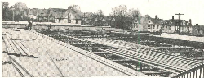
Truscon "Ferrobord" Steeldeck being used with "Clerespan" Joists for ideal fire-resistant roof construction.
