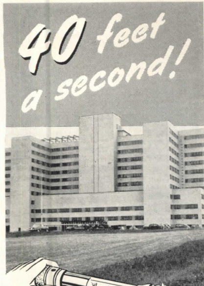
VA Hospital, Omaha, Nebraska. Architects and engineers: Ellerbe & Co., and Leo A. Daly & Co.
