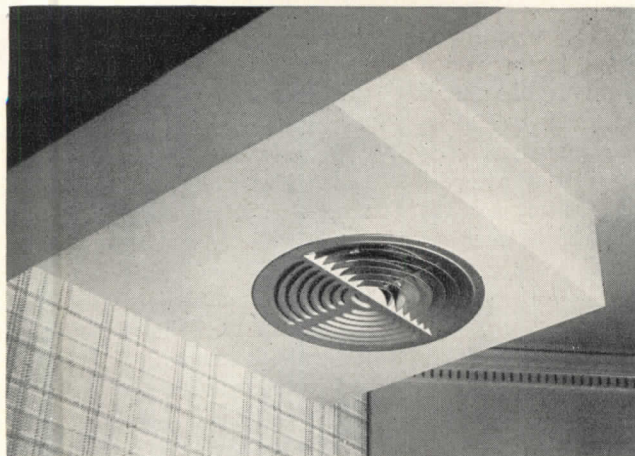
High pressure diffuser (left) uses compact ducts which may be placed in closets or in corners, as shown in construction photos above and below left
