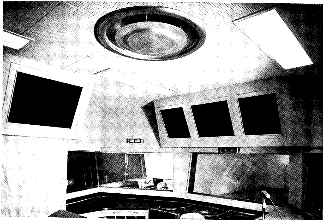
Control Room: Radio Station WFDR, New York, N. Y. Architect: Robin and Vogel, New York, N. Y. Engineer: Fred L. Moesel Associates, New York, N. Y. Mechanical Contractor: The J. M. Fink Co., New York, N. Y.
