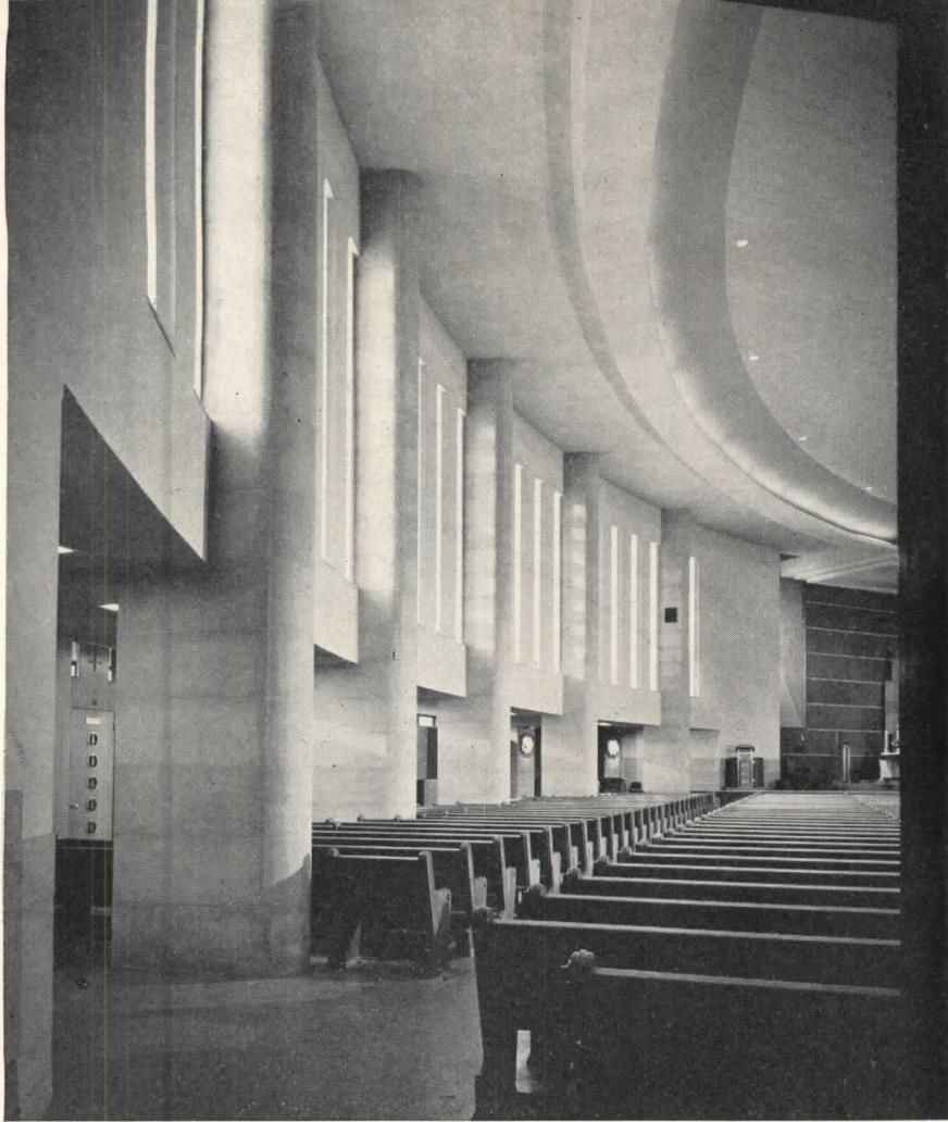
The masonry pier structure is surfaced outside with Indiana limestone, inside with Winona stone and integrally colored plaster. Heat is supplied by radiant warm air floor panels
