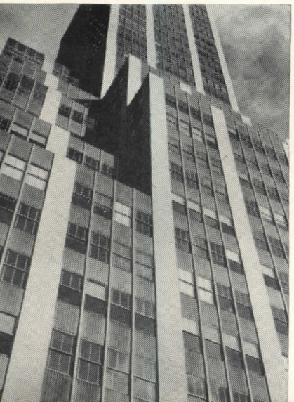
Aluminum mullions accent the vertical lines, blend with aluminum windows and spandrels.
