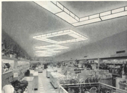
20% MORE LIGHT! This department store MODULE installation delivers 60 footcandles. To obtain the same light output with ordinary fixtures, 20% more units would be needed.
