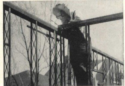
Direct Saving of 50% over masonry realized in the construction of these multiple-story apartment dwellings in Shorewood, Wisc.
