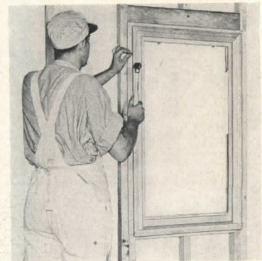
Metal window unit has wood surround for easy installation
