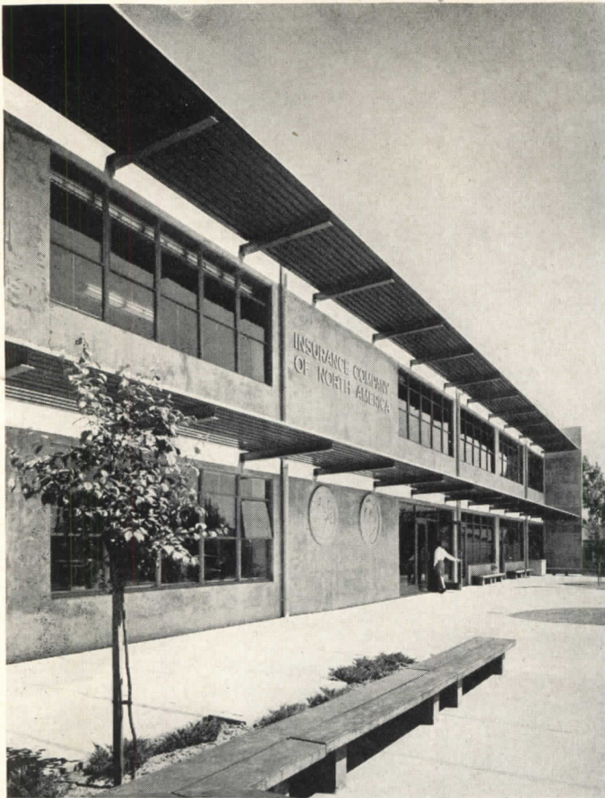
Simple, inexpensive sunshades on the southeast facade give protection against sky glare and solar heat, even though with this orientation full protection is impossible
