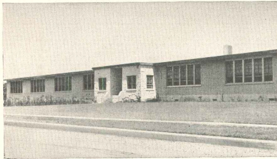
In San Antonio, the Esther Perez Carvajal School is constructed of Stran-Steel Framing. Percy W. and J. Clyde Williams, architects.
