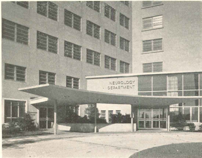
Entrance canopy serves a double entrance — outpatient department on the left, main lobby entrance at the right
