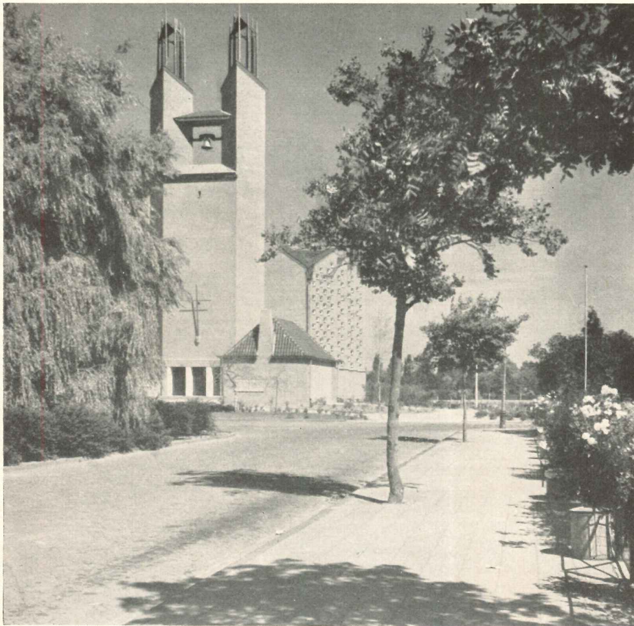
Front of church is completely closed, contrasting pleasantly with window-studded walls on other three sides. Bell hangs free between the towers, far above church doors
