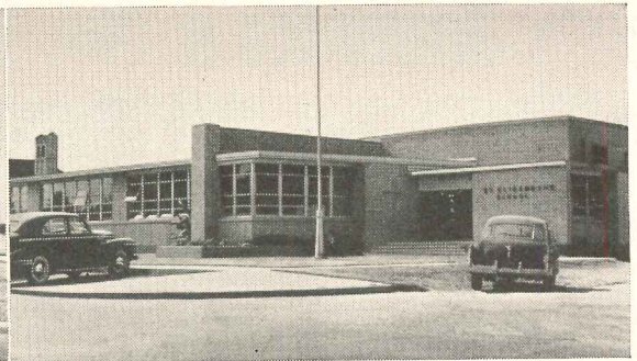
Stran-Steel Framing was used in walls, roof and partitions in the St. Elizabeth School, Alice, Texas. Wade, Gibson & Martin, architects.
