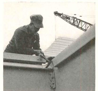
Typical scenes in assembly process: at left, living-dining unit is being lowered in place over foundation; center, kitchen-utility unit is swung into place; right, workman tightens fittings connecting two units
