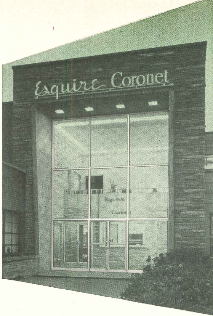
Esquire Coronet publications building in Boulder, Colorado. A striking treatment of an entrance unit featuring Kawneer doors and mullion construction. Architect—Ralph Stoetzel.
