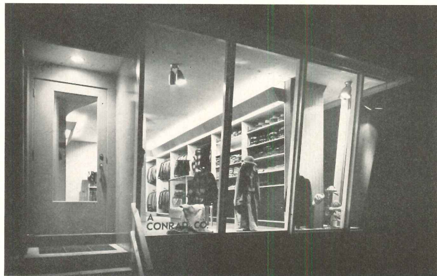
E. A. Conrad Co., Beverley, Mass.; Constantin A. Pertzoff and Louisa V. Conrad, Associated Architects. Shop serves two age groups, each with separate sales areas. Slanting bay windows reduce sky reflection
