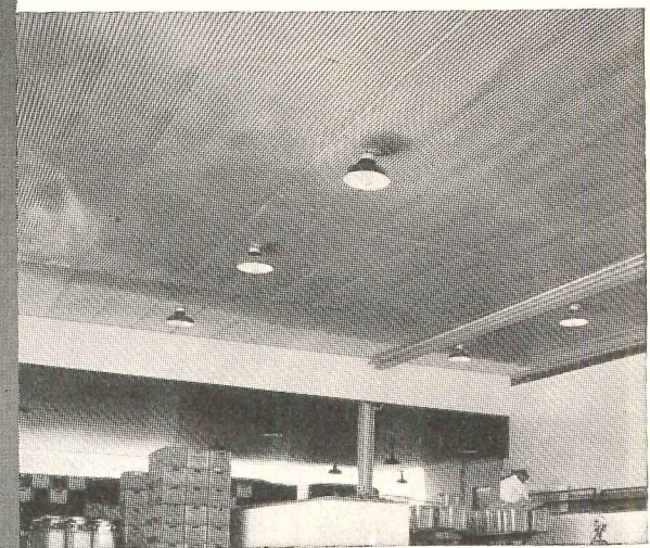
Kaiser Aluminum Roofing is effectively used as a ceiling liner in a Golden State Dairy building at Van Nuys, California. Because it is so easy to clean, aluminum contributes to maximum sanitation. Because it's solid aluminum—not clad or veneered—this ceiling is highly resistant to rust and corrosion. Never requires painting. Virtually maintenance-free. Strong—durable—lasts for years. And because aluminum is so light in weight, it is far easier to install.
