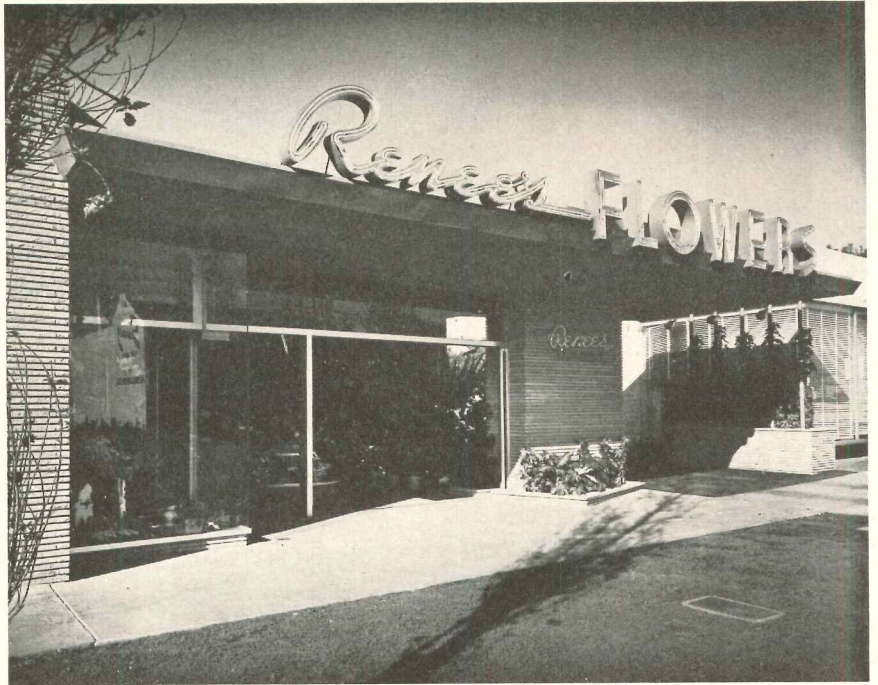
Above: Renee's Flower Shop, Beverly Hills, Calif.; Paul R. Williams, Architect; Robert Kliegman, Associate Architect. Overhang shades front, controls glare. Outdoor planting boxes help identify shop
