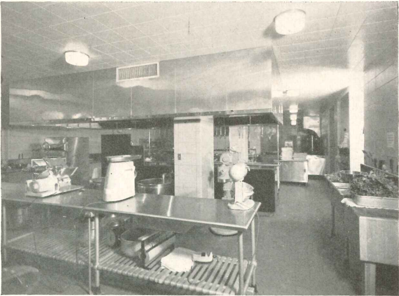
Main kitchen, in basement
