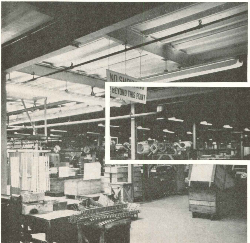
Fixtures in the foreground direct 10 per cent of their light onto the ceiling to help reduce brightness contrasts. Note, in comparison, the spotty effect of the fixtures in the inset section of the photo where all light is directed downward
