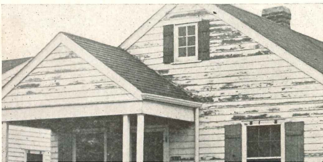
Below: note cracking and peeling on both the heated wall of the house and also on the unheated porch gable, indicating that a short-lived paint was applied. The house was repainted about 18 months before the picture was taken
