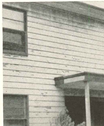
Below: note cracking and peeling on both the heated wall of the house and also on the unheated porch gable, indicating that a short-lived paint was applied. The house was repainted about 18 months before the picture was taken
