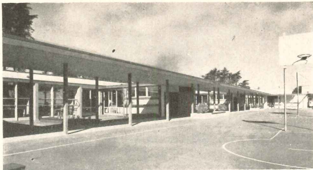
Above: Katherine Delmar Burke School, San Francisco, was a merit award winner. Architects are Donald Beach Kirby and Thomas B. Mulvin. Below: Only library building among the award winners. Hayward Public Library, John Carl Warnecke, architect
