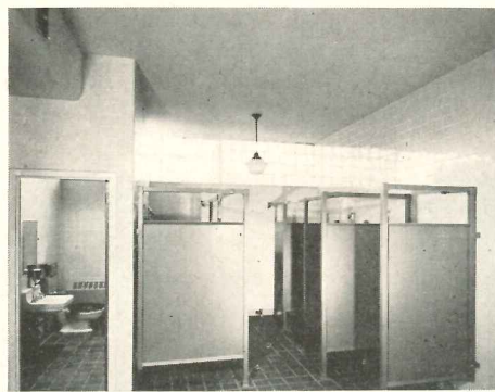
Corridors and toilets have full ceramic tiled walls; acoustic ceilings are used throughout. Above, corridor leading to lower grades; through door at end, one enters the large Kindergarten room shown on the facing page. In this room, corridor width is added to room dimension, while the clerestory windows are uninterrupted. Below, main lobby, from which are reached upper grades and administrative offices; lower grades; and multipurpose room
