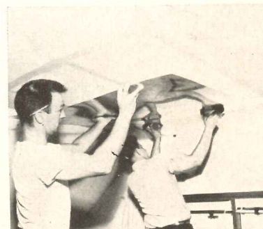
Electric radiant heating panel
