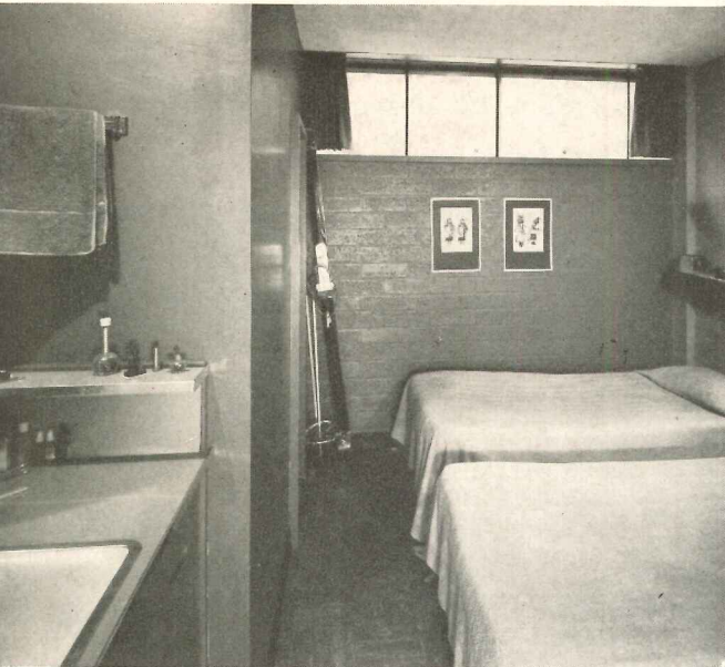
Bedroom; utility wall at left
